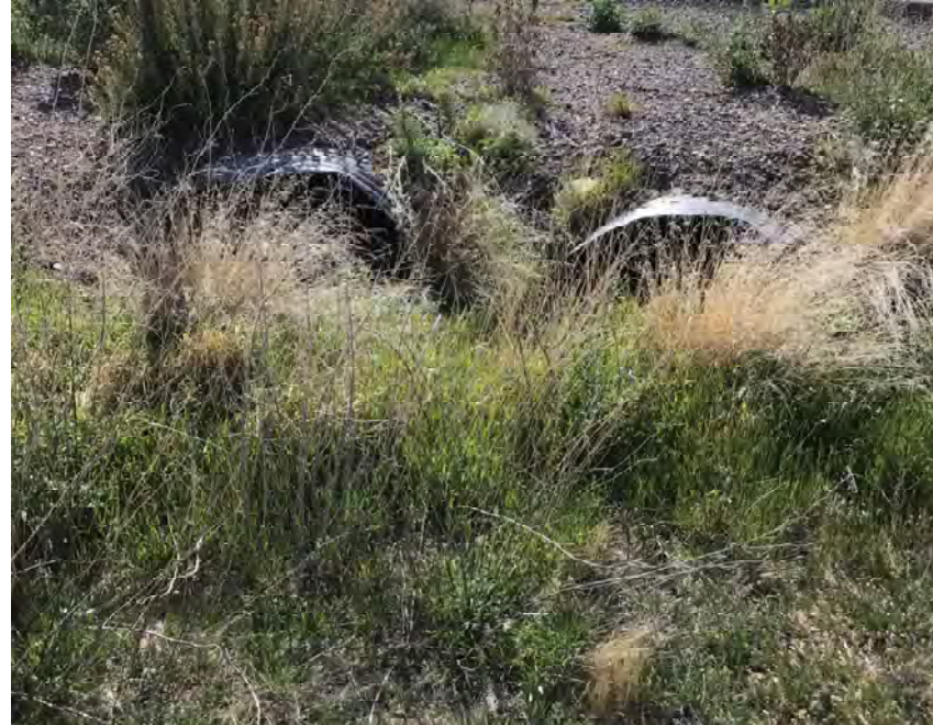
CULVERT #330 INLET (2) - 43" X 27" CMP ARCH STA 1317+00
