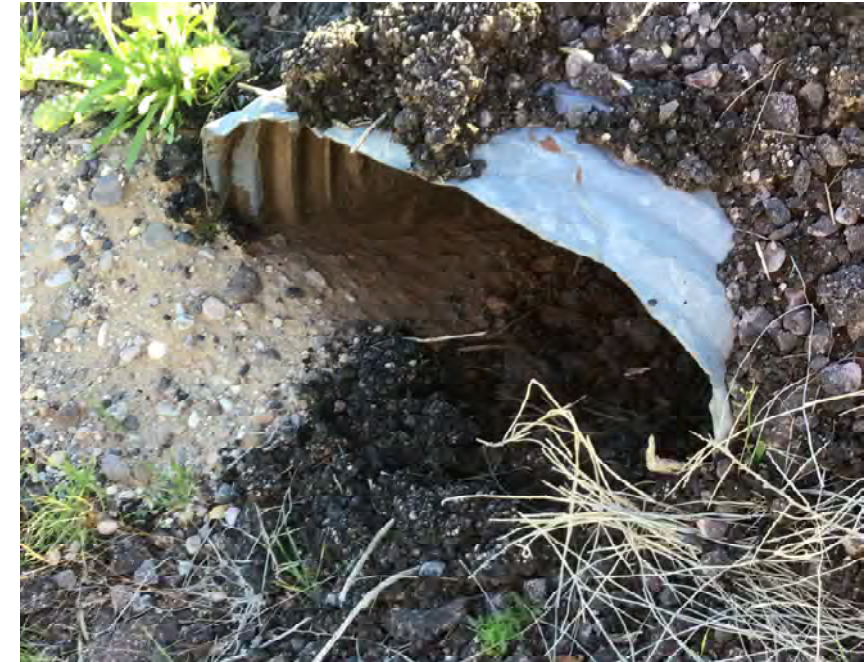
CULVERT #135 INLET 30" CMP STA 1097+00
