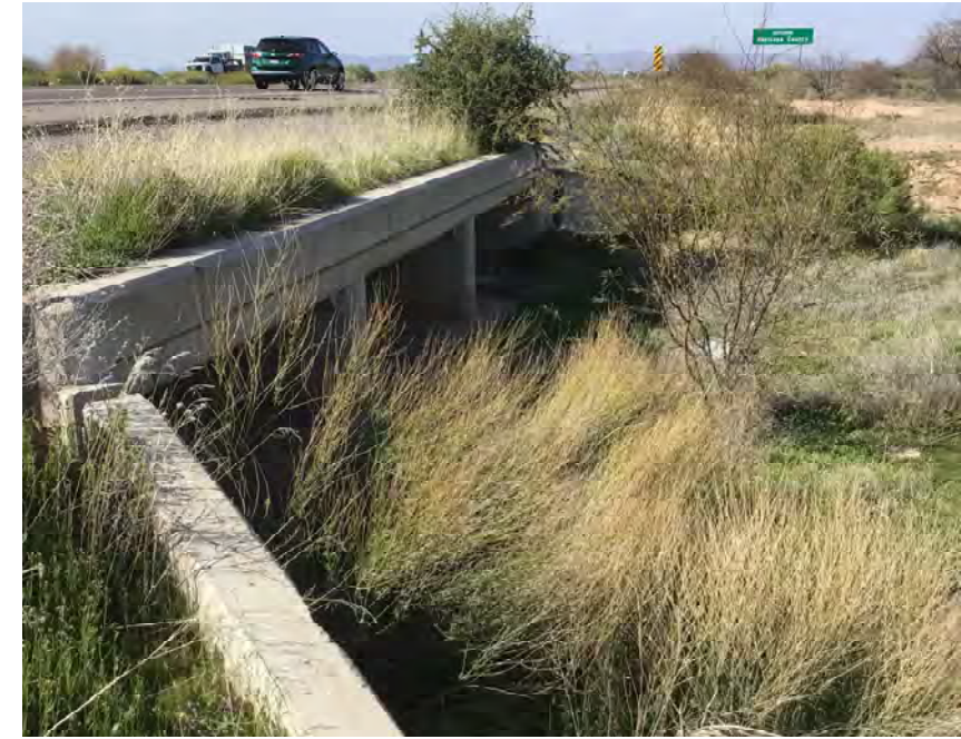
CULVERT #260 INLET BOX CULVERT 3- 10' X 3' STA 1244+20
