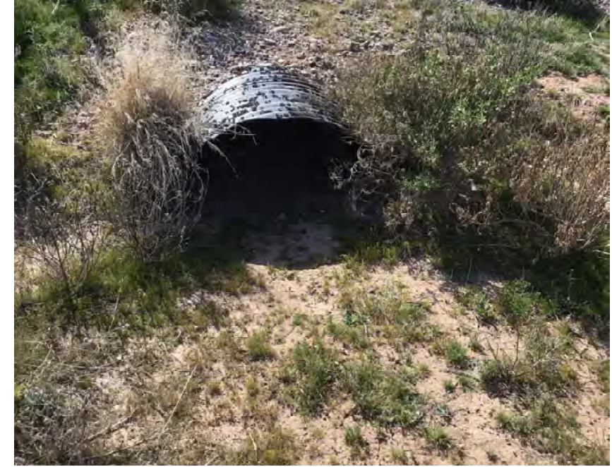
CULVERT #240 INLET 36" X 22" CMP ARCH STA 1233+00
