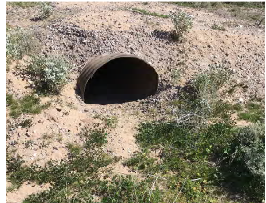
CULVERT #185 OUTLET 36" X 22" CMP ARCH STA 1151+00
