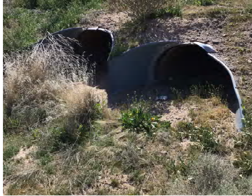
CULVERT #340 INLET (2) - 43" X 27" CMP ARCH STA 1329+00
