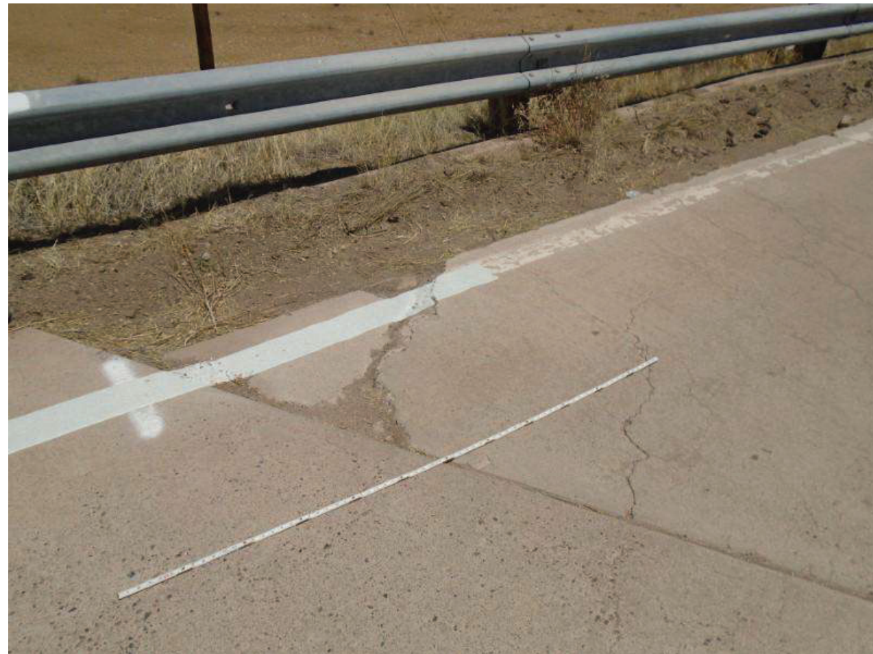
File Name : 01216-2020-05-31-Photo-11.JPG Description : Local Settlement, NE Approach Roadway, LN
