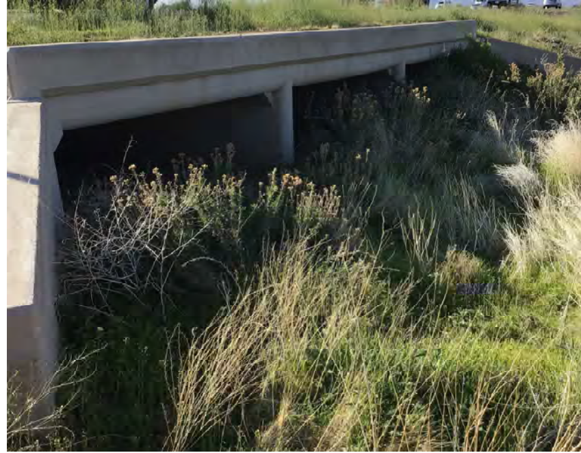
CULVERT #160 INLET BOX CULVERT 3- 10' X 3' STA 1127+00
