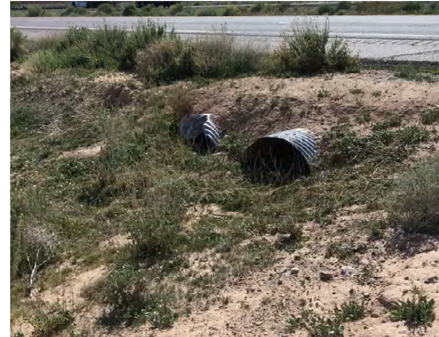
CULVERT #315 INLET (2) - 43" X 27" CMP ARCH STA 1297+00
