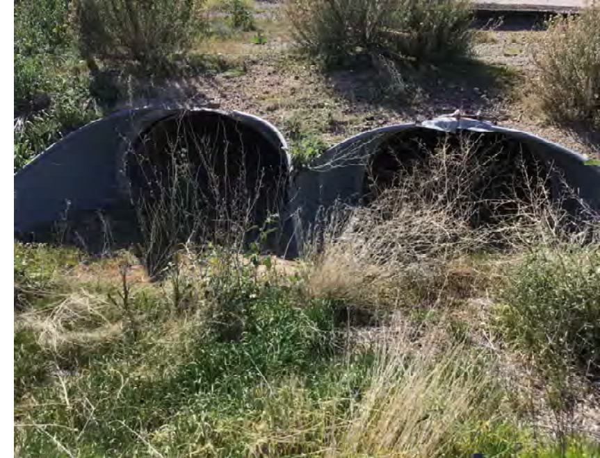
CULVERT #335 INLET (2) - 43" X 27" CMP ARCH STA 1323+00
