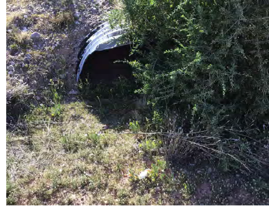
CULVERT #155 INLET 29" X 18" CMP ARCH STA 1124+50
