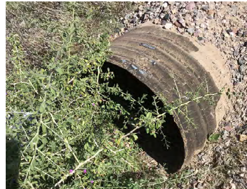
CULVERT #155 OUTLET 29" X 18" CMP ARCH STA 1124+50
