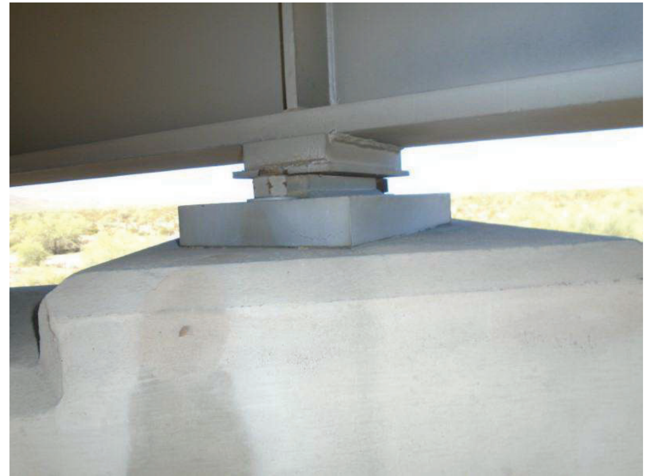
File Name : 01150-2020-05-31-Photo-14.JPG Description : Pier 2, Typical Bearing Condition, LSW
