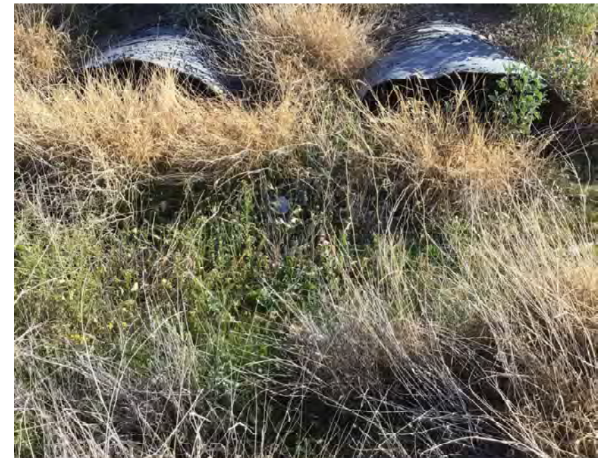
CULVERT #300 OUTLET (2) - 43" X 27" CMP ARCH STA 1285+00
