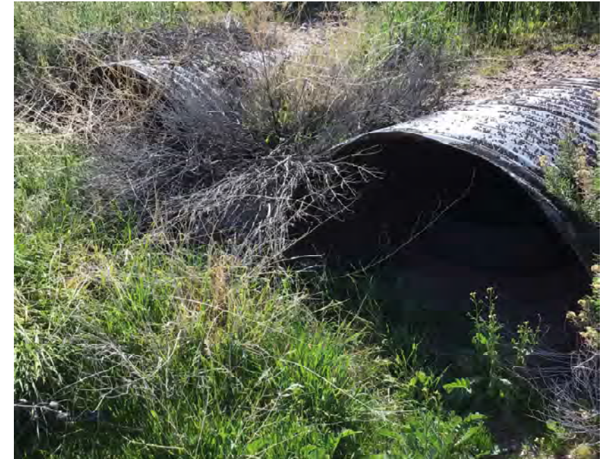
CULVERT #375 INLET (2) - 58" X 36" CMP ARCH STA 1378+00
