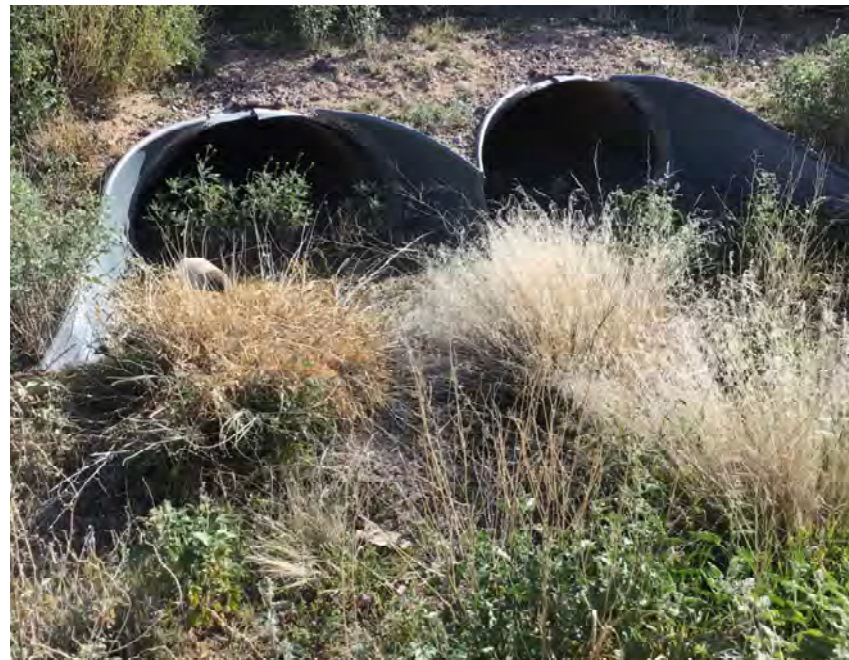
CULVERT #330 OUTLET (2) - 43" X 27" CMP ARCH STA 1317+00
