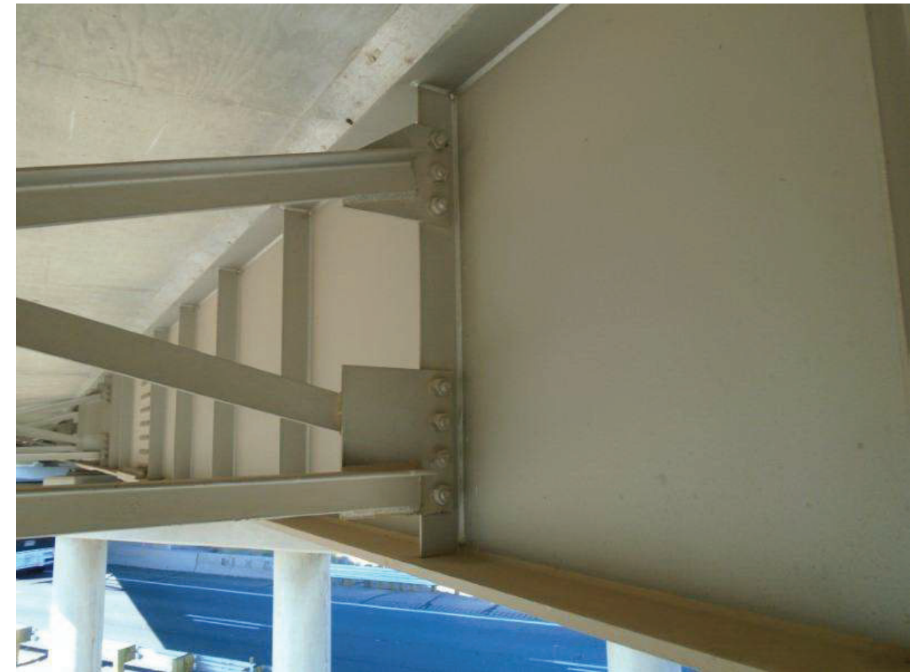
File Name : 01215-2020-05-31-Photo-17.JPG Description : Typical Diaphragm Connection
