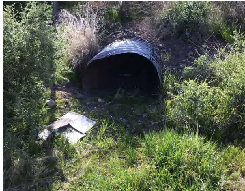
CULVERT #225 INLET 30" CMP STA 1211+00
