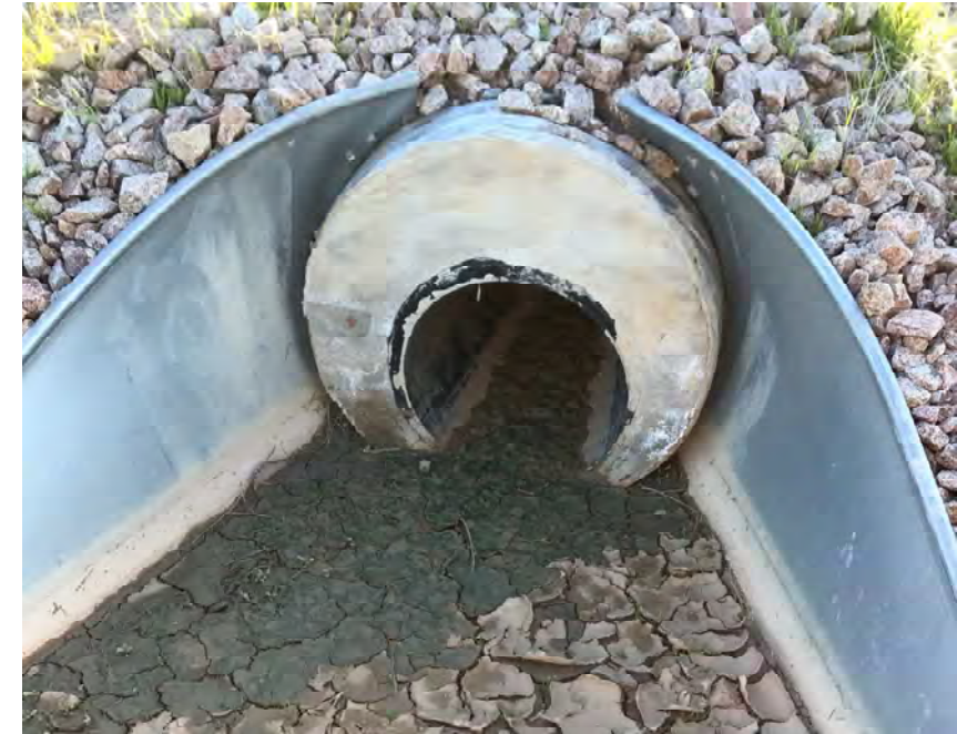
CULVERT #65 INLET 18" CMP STA 1008+10
