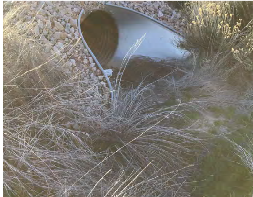
CULVERT #50 INLET 30" CMP STA 986+00
