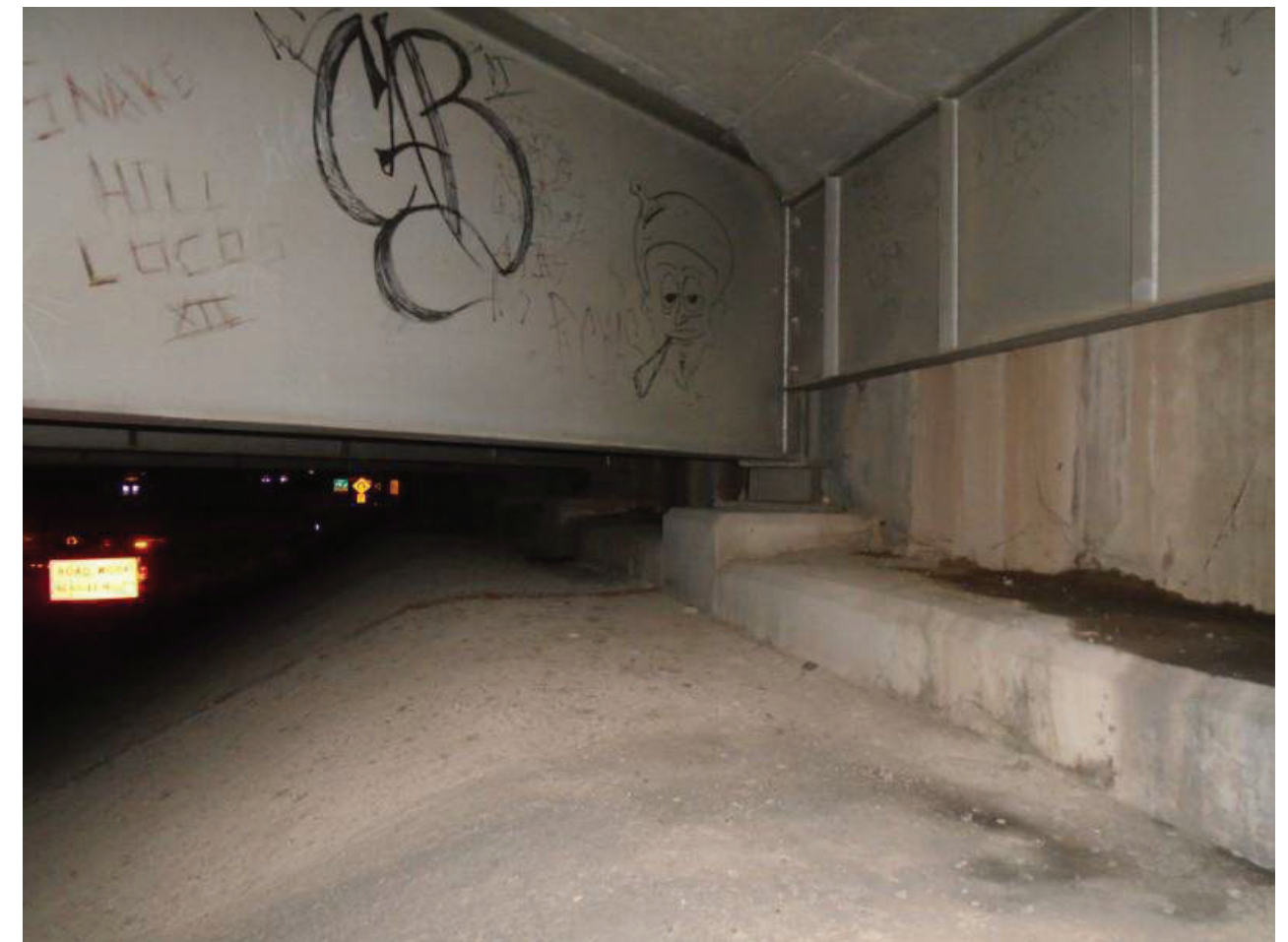
File Name : 01214-2020-05-31-Photo-19.JPG Description : South Abutment, LSE
