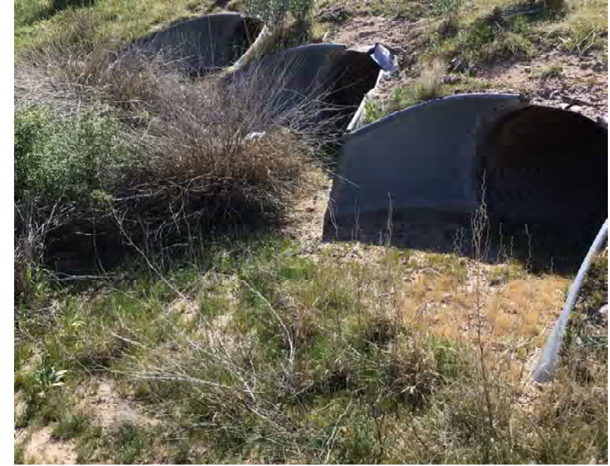
CULVERT #345 INLET (3) - 43" X 27" CMP ARCH STA 1335+00
