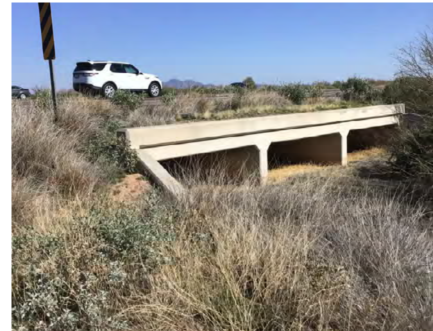
CULVERT #270 OUTLET BOX CULVERT 3- 10' X 3' STA 1253+00
