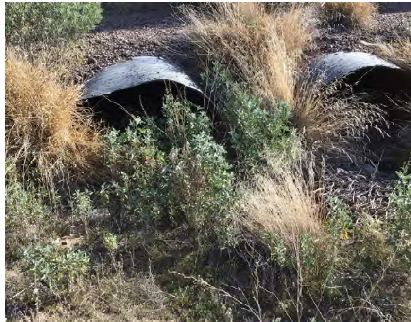
CULVERT #320 OUTLET (2) - 50" X 31" CMP ARCH STA 1305+20
