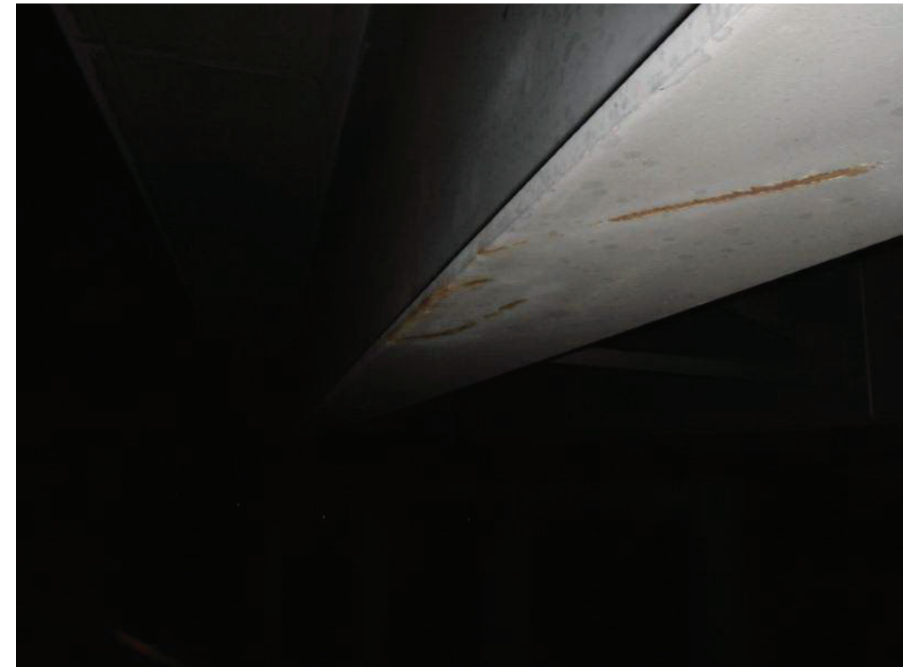
File Name : 01150-2020-05-31-Photo-20.JPG Description : Scrape Marks, Bottom Flange, Girder 4, Over WB Right Lane, LS
