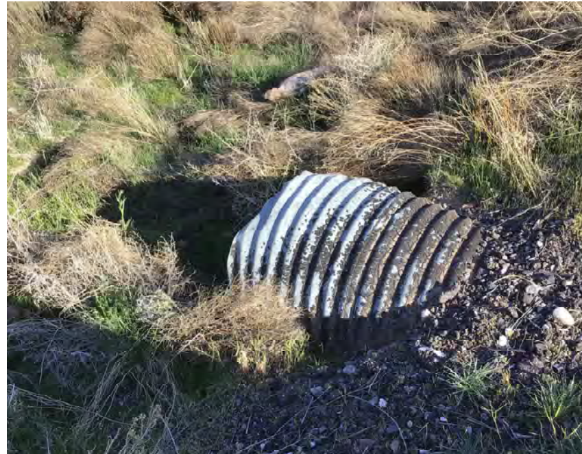
CULVERT #110 INLET 30" CMP STA 1064+00
