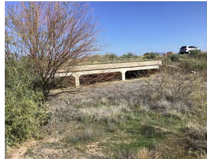
CULVERT #260 OUTLET BOX CULVERT 3- 10' X 3' STA 1244+20
