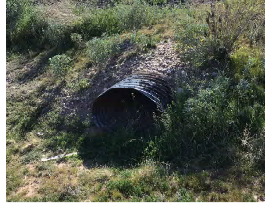
CULVERT #185 INLET 36" X 22" CMP ARCH STA 1151+00
