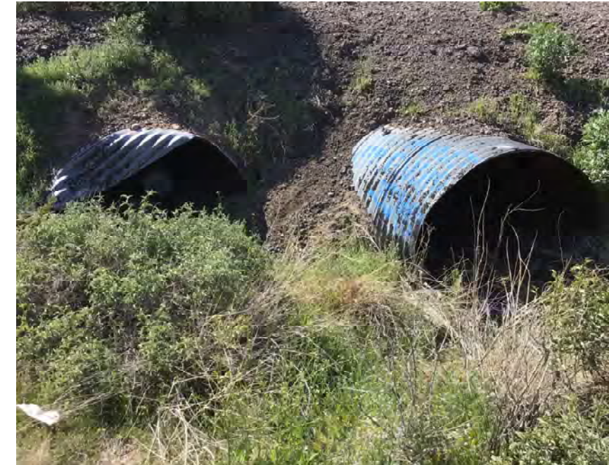
CULVERT #435 INLET (2) - 58" X 36" CMP ARCH STA 1461+83
