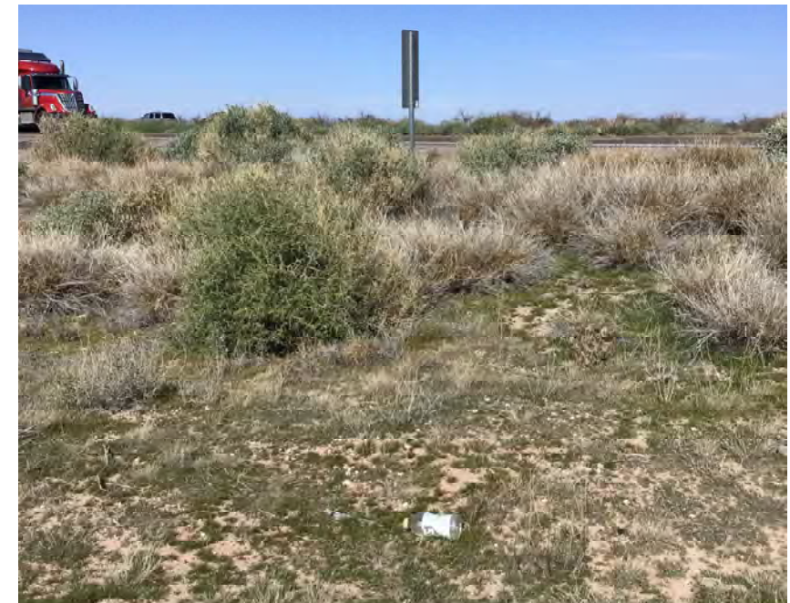
CULVERT #240 OUTLET 36" X 22" CMP ARCH STA 1233+00
