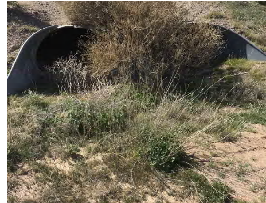
CULVERT #325 INLET (2) - 43" X 27" CMP ARCH STA 1311+00
