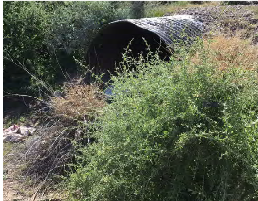
CULVERT #370 INLET (2) - 58" X 36" CMP ARCH STA 1371+00
