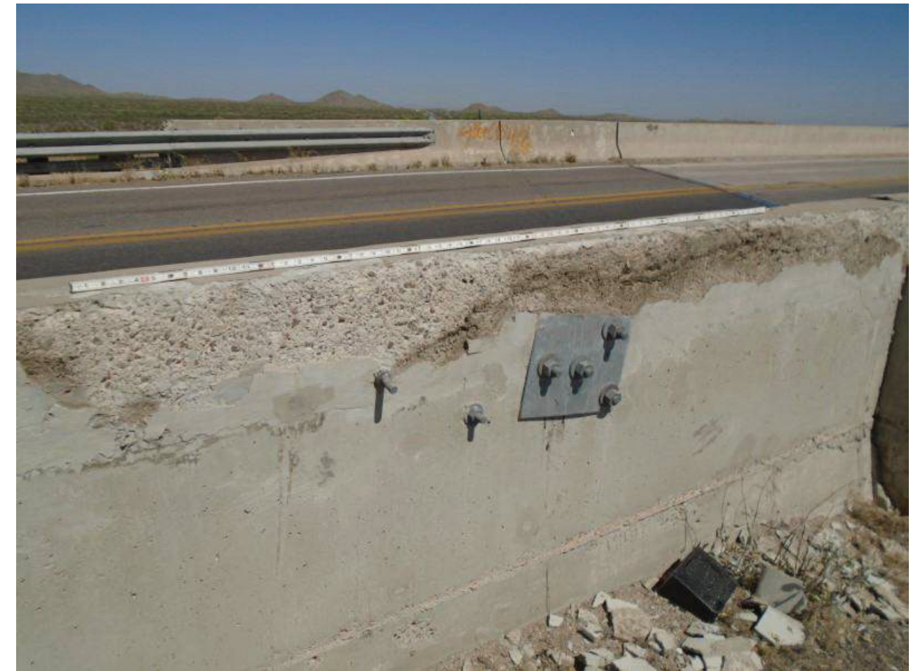
File Name : 01151-2020-05-22-Photo-9.JPG Description : Scaling, SE Approach Transition Railing, LW
