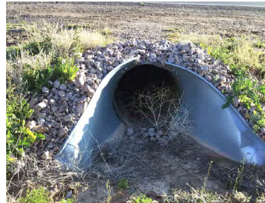
CULVERT #65 OUTLET 30" CMP STA 1008+10
