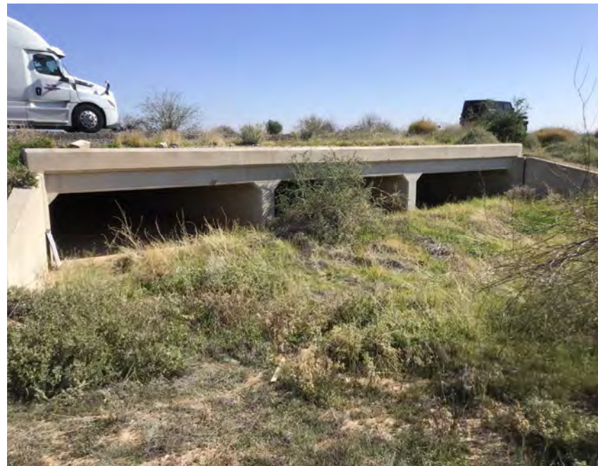
CULVERT #160 OUTLET BOX CULVERT 3- 10' X 3' STA 1127+00
