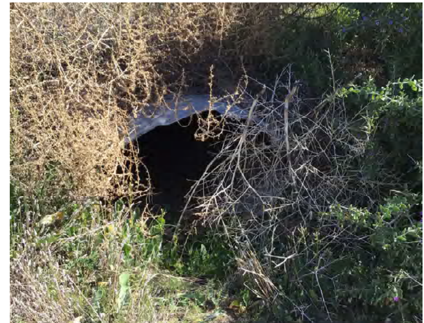
CULVERT #165 OUTLET 29" X 18" CMP ARCH STA 1130+00
