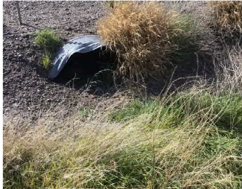
CULVERT #305 INLET (2) - 43" X 27" CMP ARCH STA 1291+00
