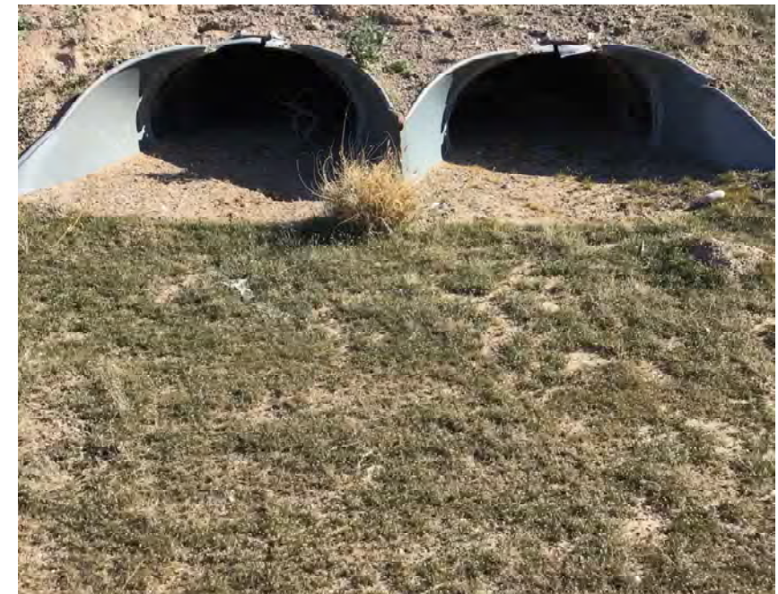
CULVERT #355 OUTLET (2) - 43" X 27" CMP ARCH STA 1347+00
