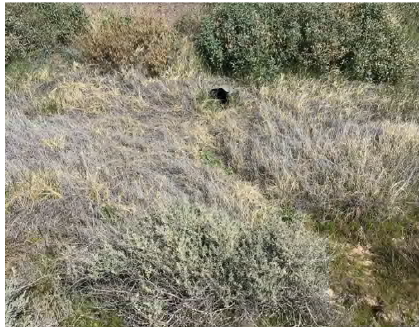
CULVERT #245 OUTLET 29" X 18" CMP ARCH STA 1237+00
