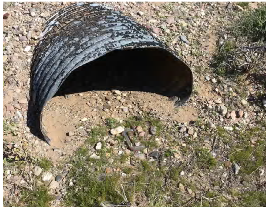
CULVERT #235 OUTLET 36" X 22" CMP ARCH STA 1224+00
