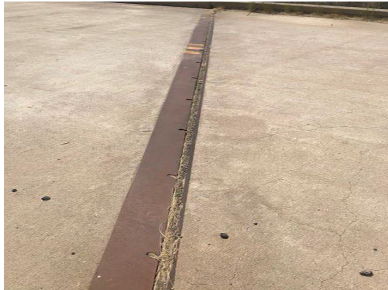
File Name : 01149-2021-05-18-Photo-5.jpg Description : Joint at W abutment
