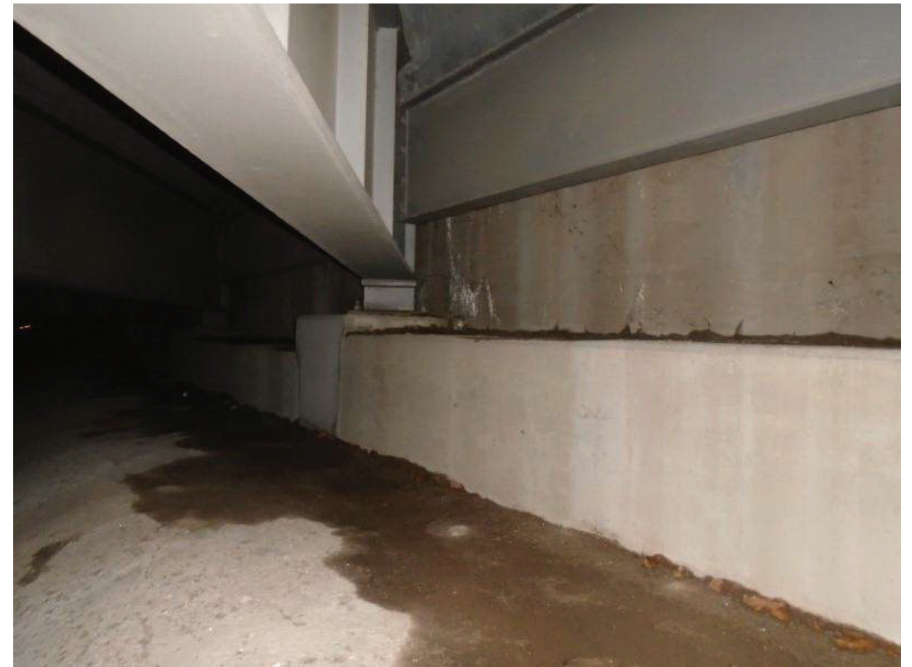
File Name : 01215-2020-05-31-Photo-9.JPG Description : North Abutment, LNW
