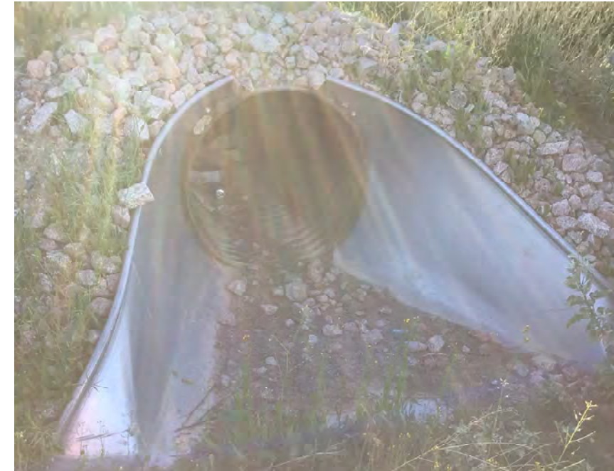
CULVERT #75 INLET 30" CMP STA 1018+00
