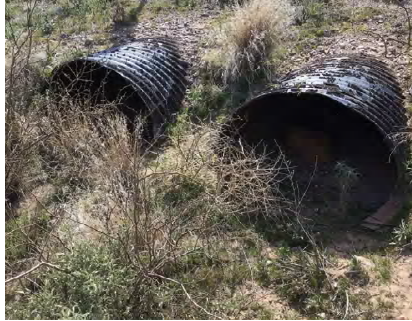
CULVERT #295 INLET (2) - 43" X 27" CMP ARCH STA 1279+00
