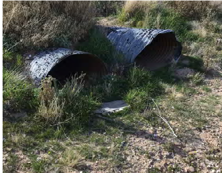
CULVERT #265 INLET (2) - 43" X 27" CMP ARCH STA 1249+00
