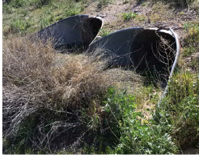
CULVERT #350 INLET (2) - 43" X 27" CMP ARCH STA 1341+00
