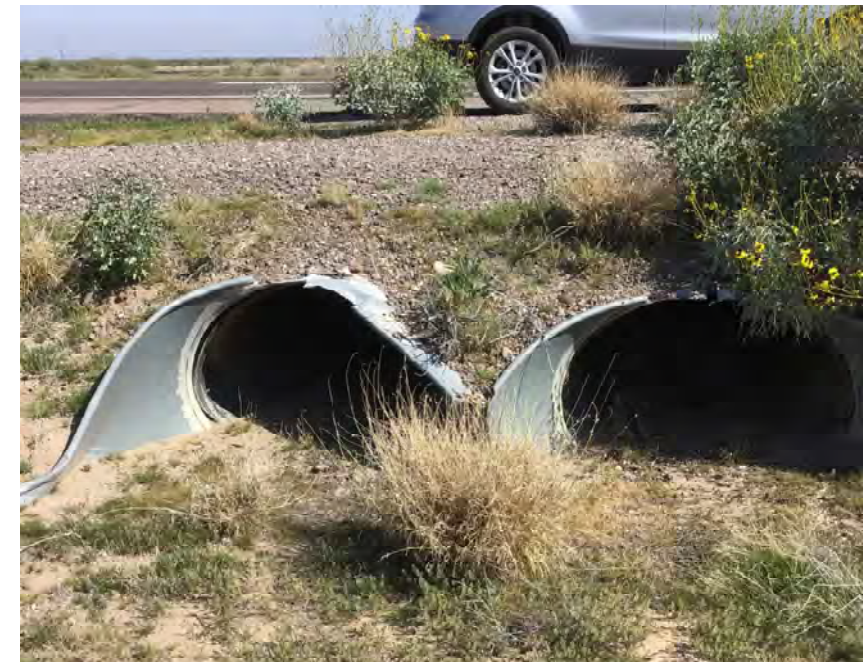
CULVERT #425 OUTLET (2) - 43" X 27" CMP ARCH STA 1435+00
