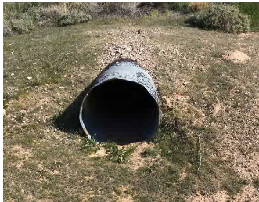
CULVERT #140 OUTLET 30" CMP STA 1105+50
