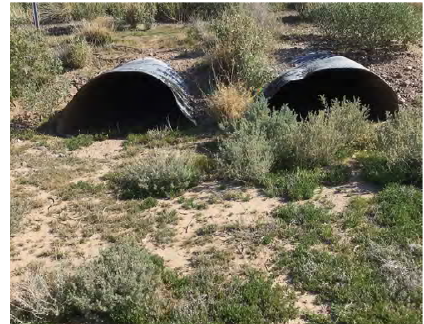
CULVERT #375 OUTLET (2) - 58" X 36" CMP ARCH STA 1378+00
