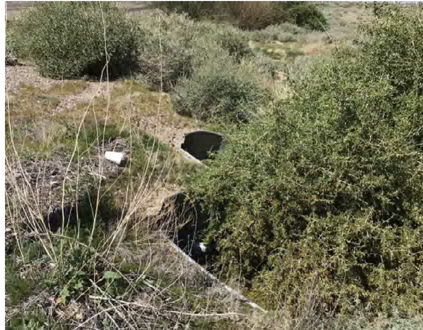
CULVERT #390 INLET (3) - 43" X 27" CMP ARCH STA 1395+00
