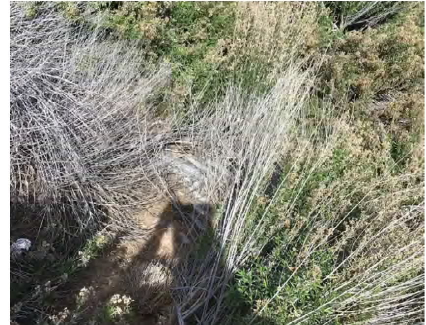
CULVERT #290 INLET (2) - 43" X 27" CMP ARCH STA 1273+00
