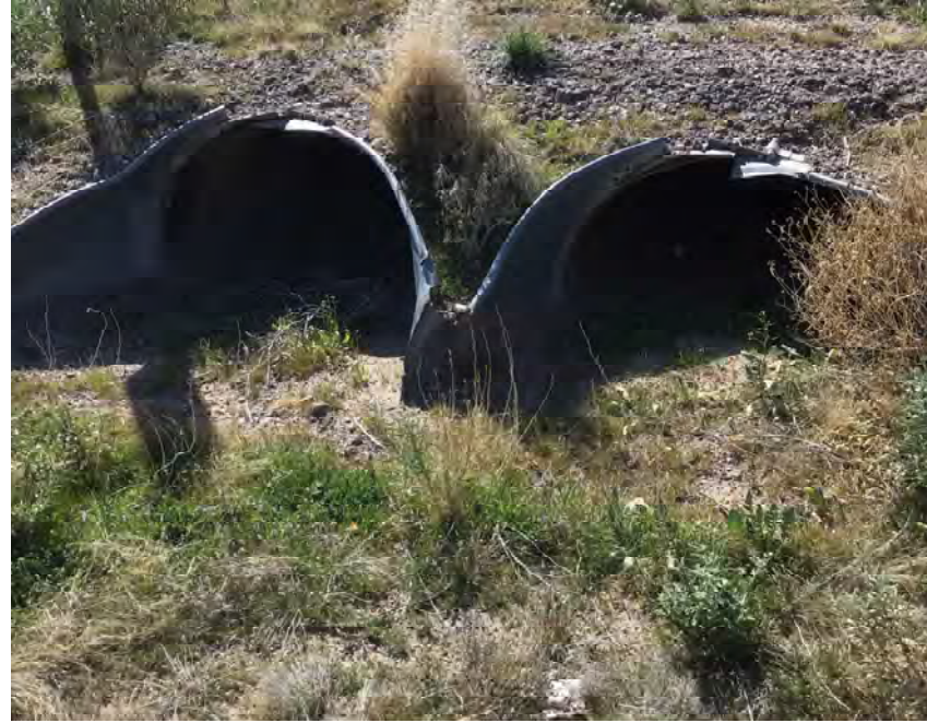
CULVERT #360 INLET (2) - 43" X 27" CMP ARCH STA 1353+00
