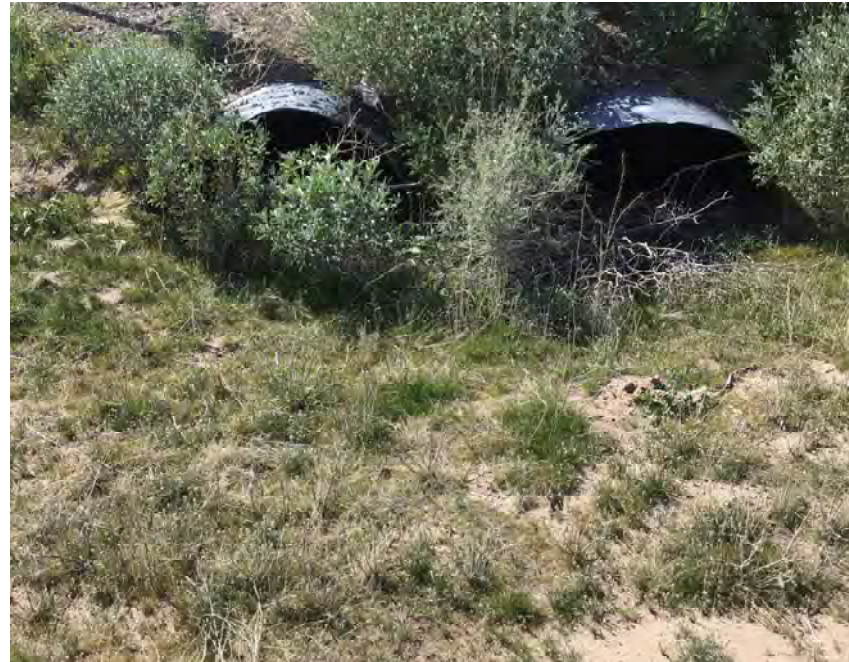
CULVERT #420 INLET (2) - 43" X 27" CMP ARCH STA 1435+00
