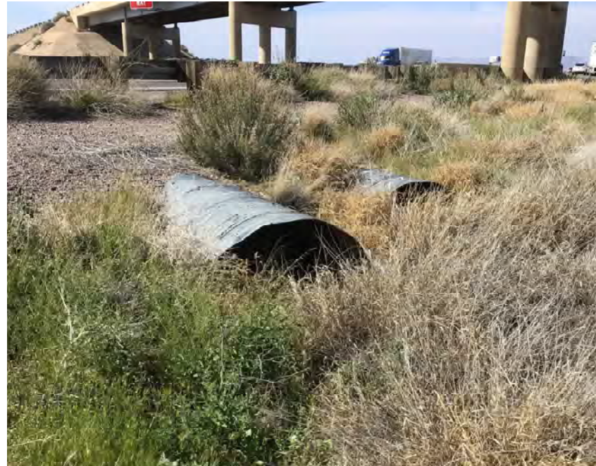
CULVERT #320 INLET (2) - 50" X 31" CMP ARCH STA 1305+20
