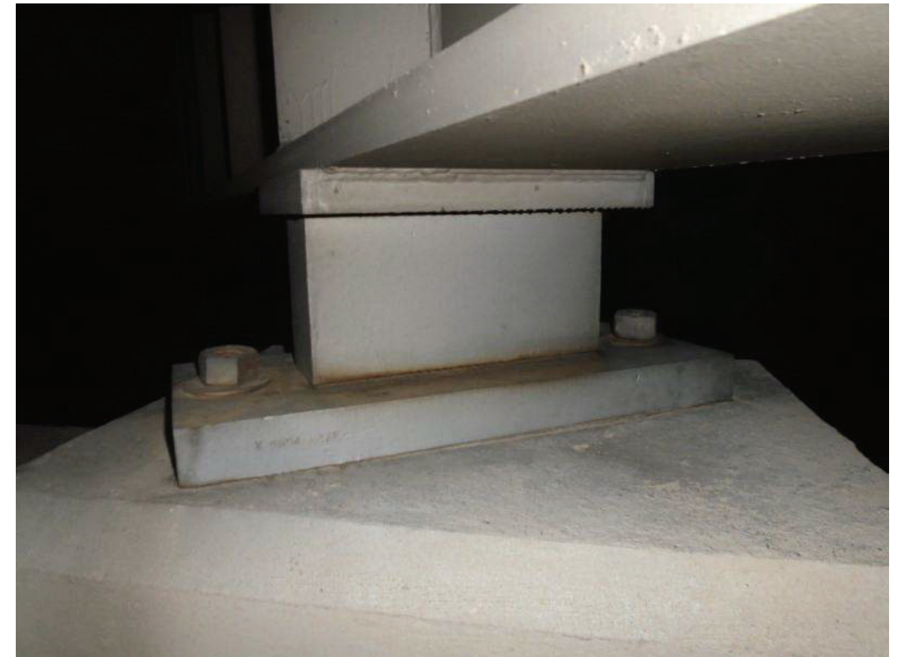
File Name : 01214-2020-05-31-Photo-13.JPG Description : Typical Bearing, Pier 1, LN
