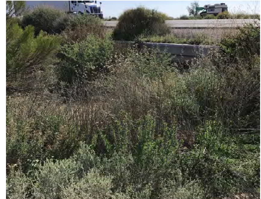
CULVERT #250 INLET BOX CULVERT 3- 10' X 3' STA 1240+33
