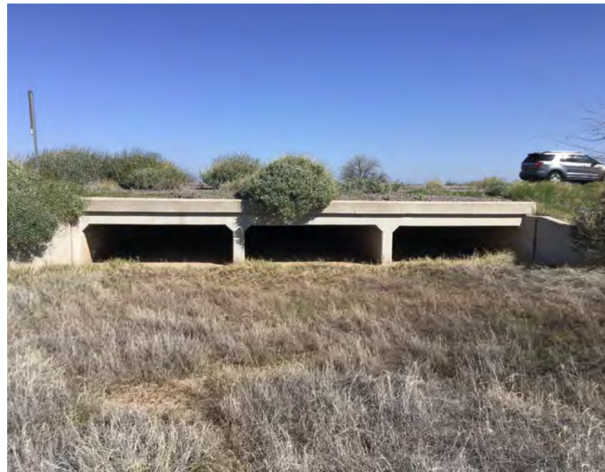
CULVERT #215 OUTLET BOX CULVERT 3- 10' X 3' STA 1202+02
