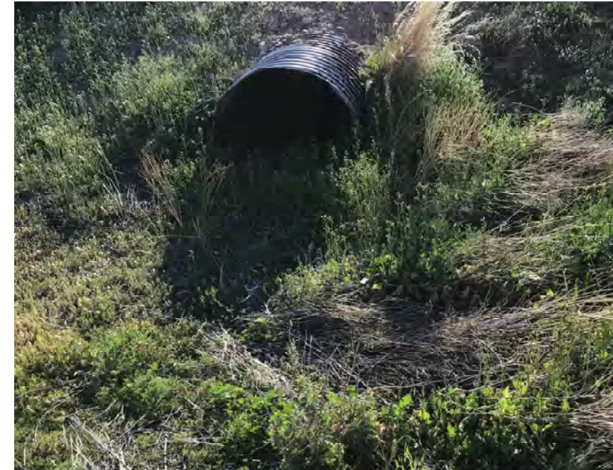
CULVERT #115 INLET 30" CMP STA 1070+00
