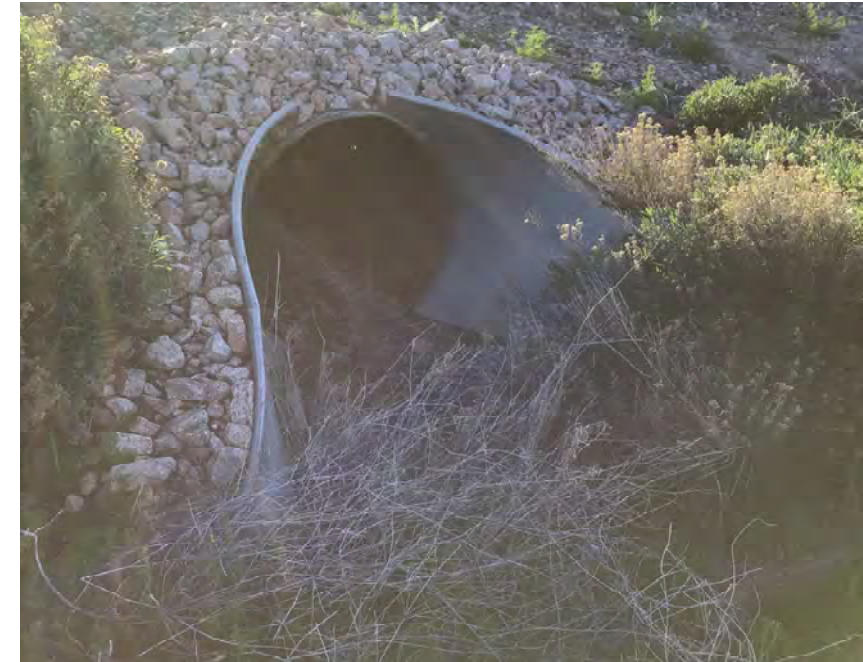
CULVERT #55 INLET 30" CMP STA 996+00
