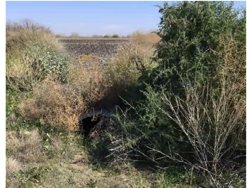
CULVERT #175 OUTLET 36" X 22" CMP ARCH STA 1136+50
