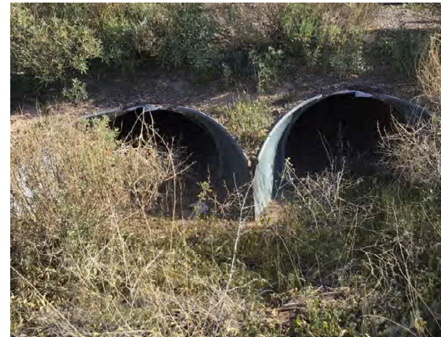
CULVERT #335 OUTLET (2) - 43" X 27" CMP ARCH STA 1323+00
