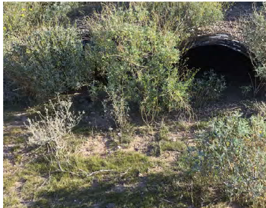
CULVERT #285 OUTLET (2) - 43" X 27" CMP ARCH STA 1267+00
