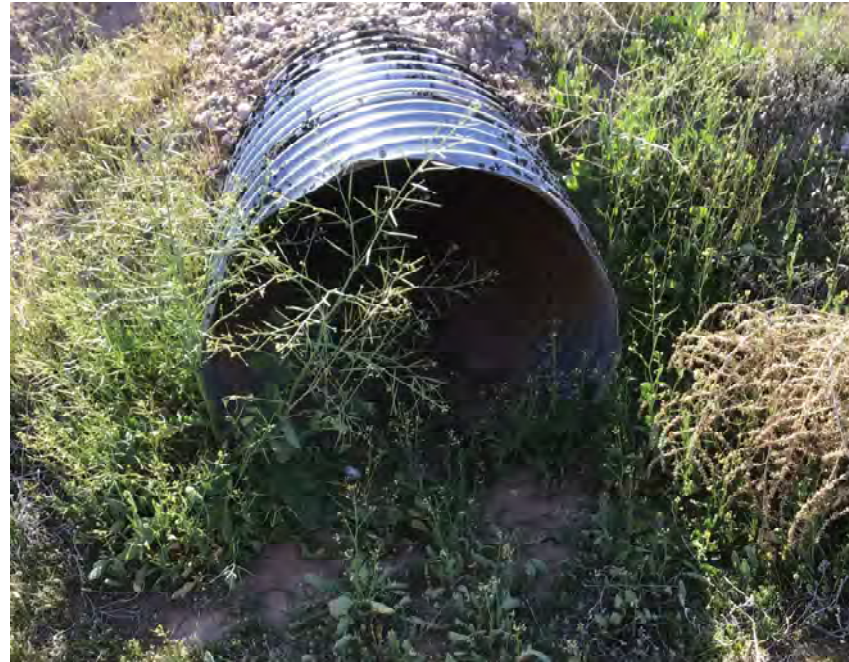
CULVERT #140 INLET 30" CMP STA 1105+50
