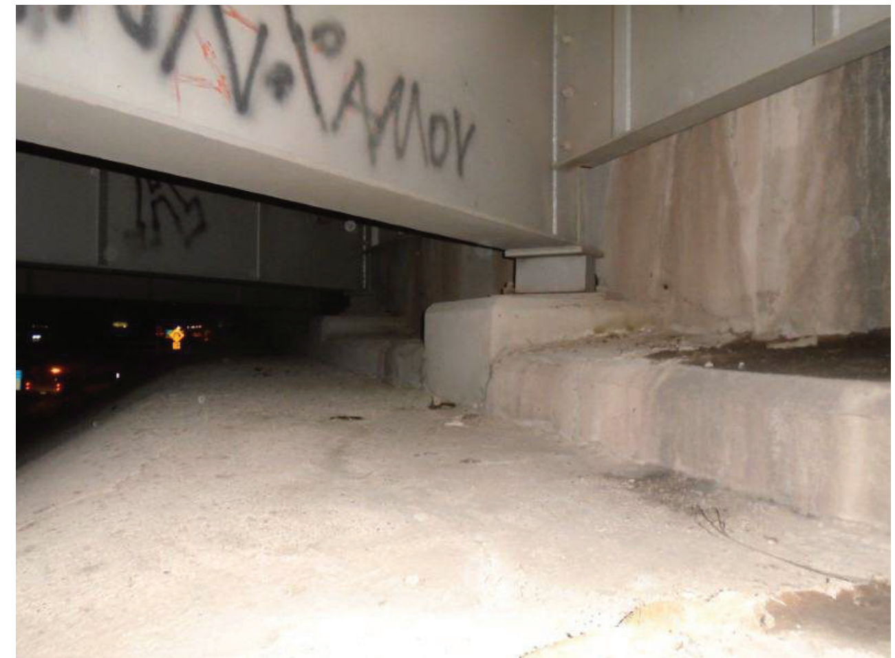
File Name : 01214-2020-05-31-Photo-11.JPG Description : North Abutment, LNE
