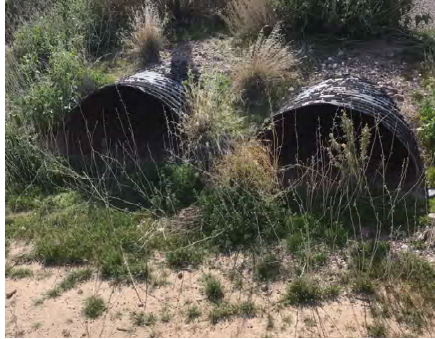
CULVERT #275 INLET (2) - 43" X 27" CMP ARCH STA 1255+00
