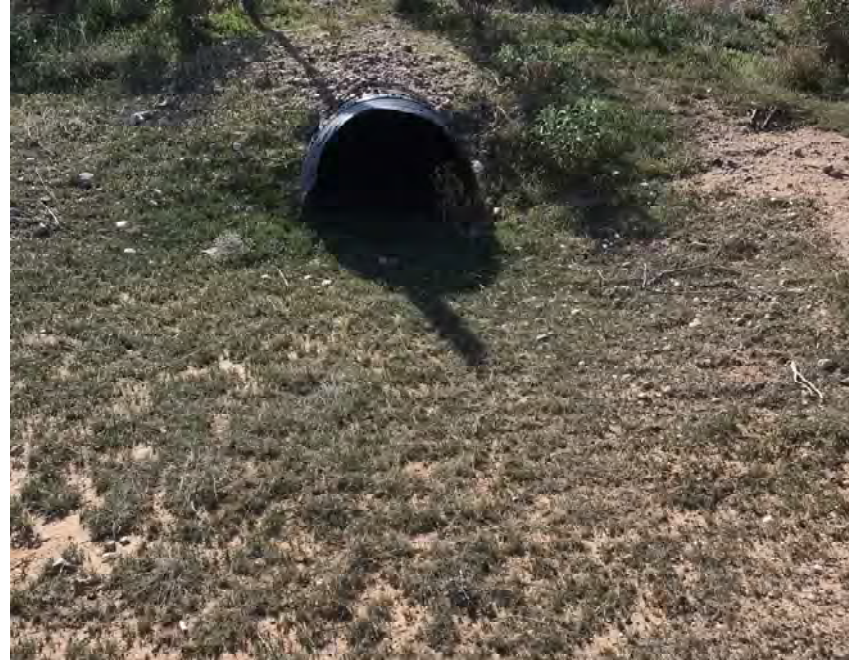
CULVERT #205 INLET 30" CMP STA 1198+50
