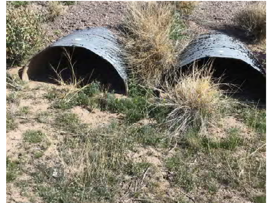
CULVERT #415 OUTLET (2) - 43" X 27" CMP ARCH STA 1429+00
