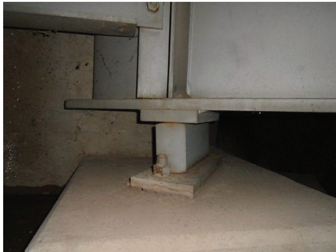
File Name : 01215-2020-05-31-Photo-10.JPG Description : Typical Bearing, North Abutment, LNE
