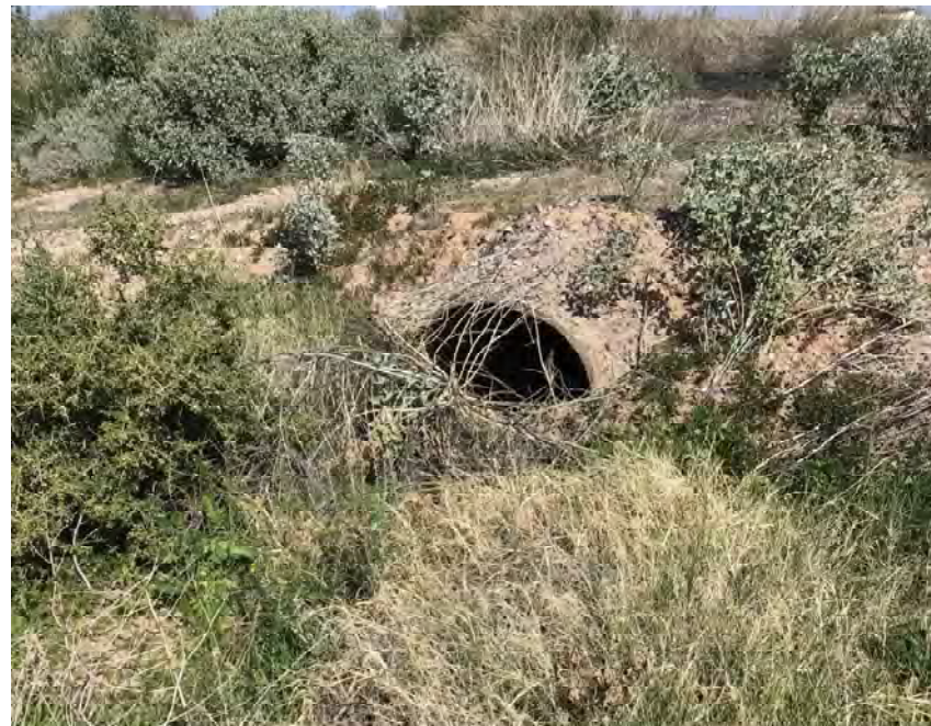
CULVERT #180 OUTLET 36" X 22" CMP ARCH STA 1143+50
