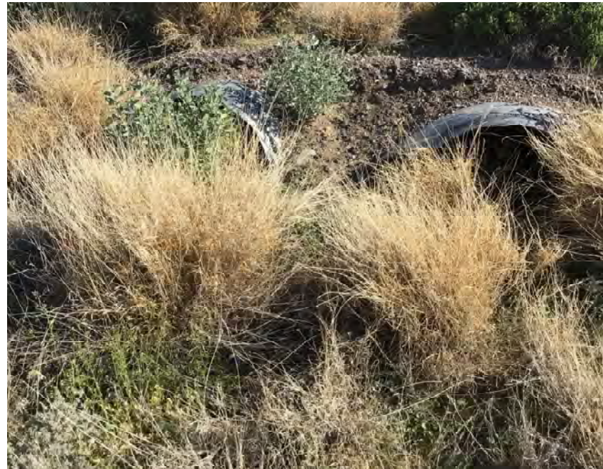
CULVERT #360 OUTLET (2) - 43" X 27" CMP ARCH STA 1353+00
