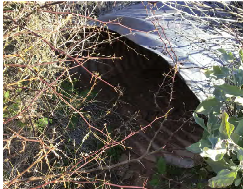
CULVERT #80 OUTLET 36" X 22" CMP ARCH STA 1029+00
