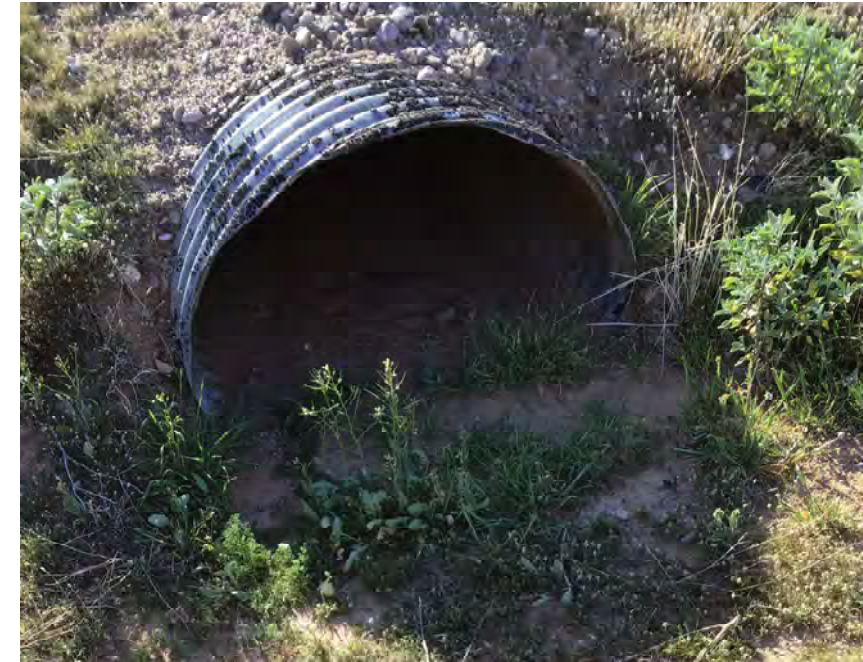
CULVERT #145 INLET 36" X 22" CMP ARCH STA 1109+00
