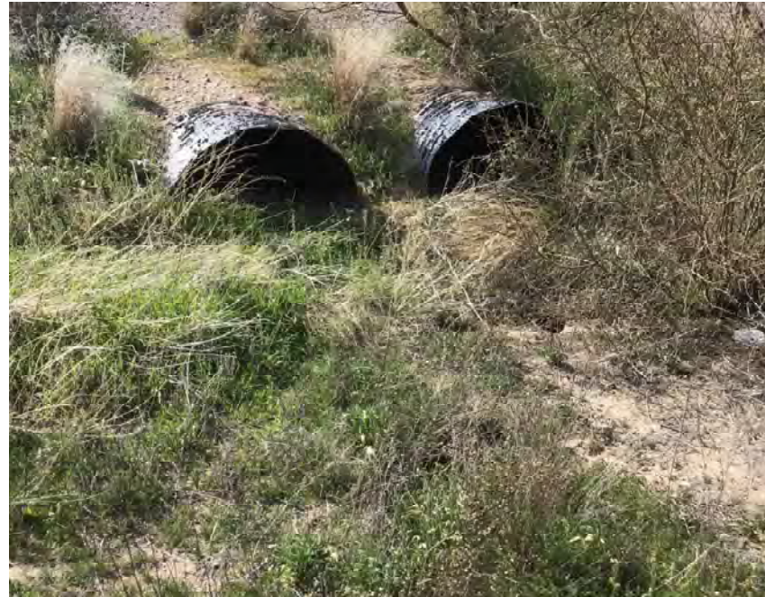
CULVERT #285 INLET (2) - 43" X 27" CMP ARCH STA 1267+00
