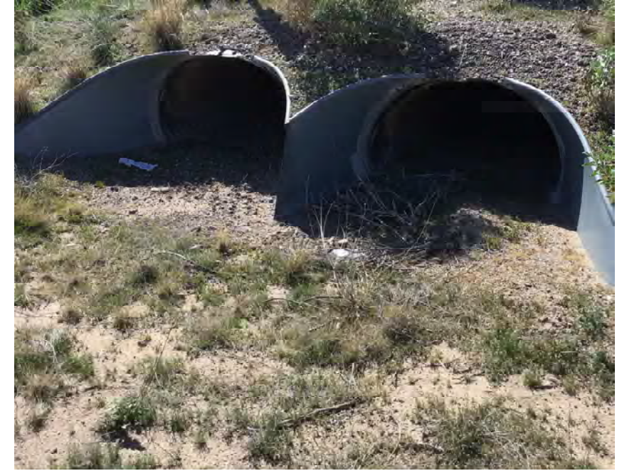
CULVERT #355 INLET (2) - 43" X 27" CMP ARCH STA 1347+00
