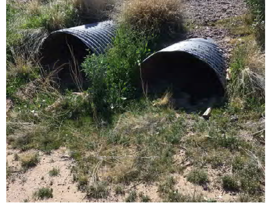
CULVERT #365 INLET (2) - 43" X 27" CMP ARCH STA 1359+00
