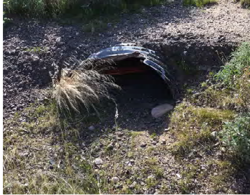
CULVERT #235 INLET 36" X 22" CMP ARCH STA 1224+00
