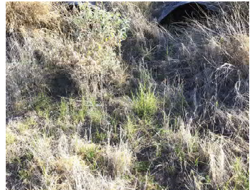
CULVERT #290 OUTLET (2) - 43" X 27" CMP ARCH STA 1273+00
