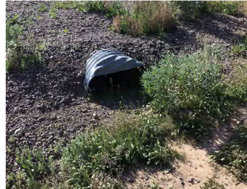
CULVERT #200 INLET 30" CMP STA 1180+00
