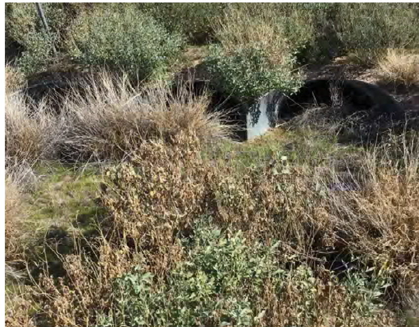
CULVERT #390 OUTLET (3) - 43" X 27" CMP ARCH STA 1395+00
