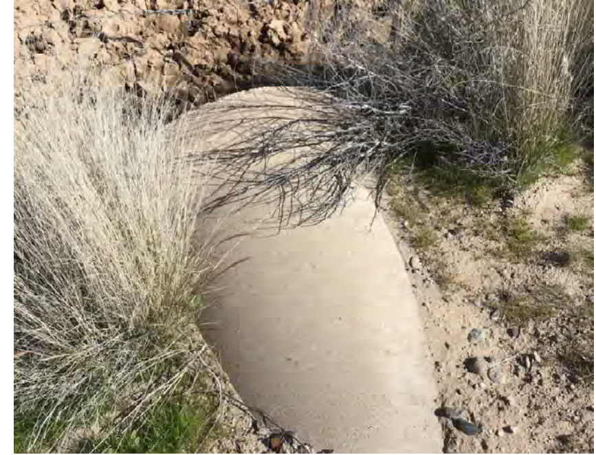
CULVERT #385 INLET 30" RCP STA 1385+44
