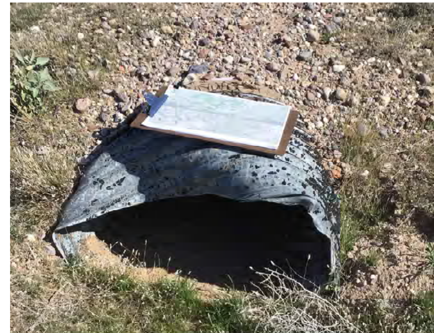
CULVERT #145 OUTLET 36" X 22" CMP ARCH STA 1109+00
