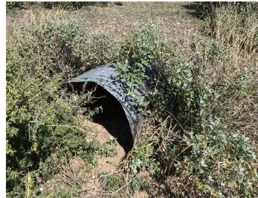
CULVERT #220 OUTLET 30" CMP STA 1208+00
