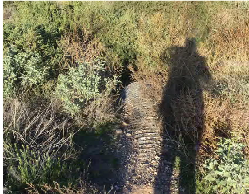
CULVERT #80 INLET 36" X 22" CMP ARCH STA 1029+00
