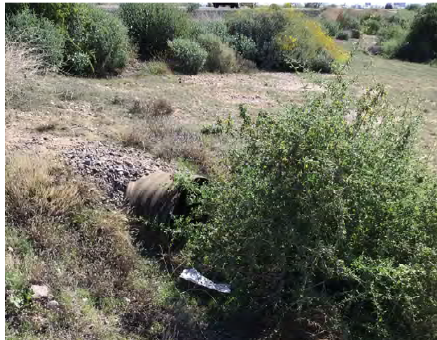
CULVERT #150 OUTLET 29" X 18" CMP ARCH STA 1117+00
