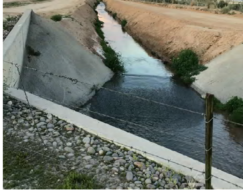
CULVERT #0 INLET BOX CULVERT 3-10' X 7' STA 915+00
