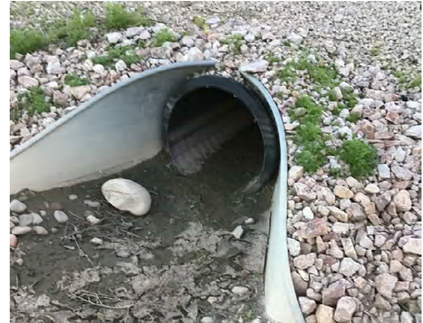
CULVERT #15 INLET 24" HDPE STA 937+00
