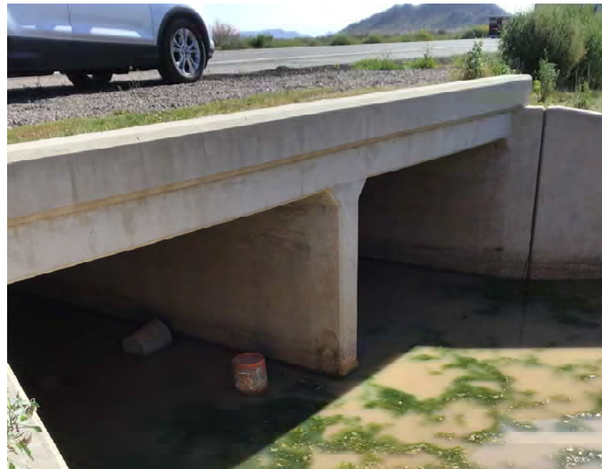
CULVERT #380 OUTLET BOX CULVERT 2-10' X 6' STA 1383+00
