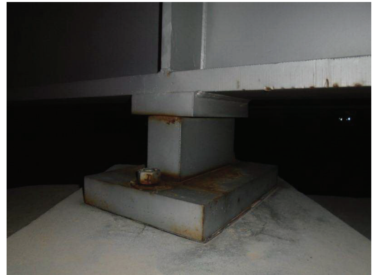
File Name : 01215-2020-05-31-Photo-11.JPG Description : Typical Bearing, Pier 4, LNE
