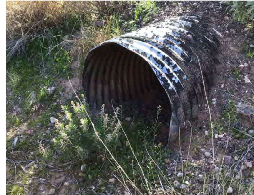
CULVERT #220 INLET 30" CMP STA 1208+00
