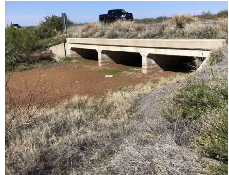
CULVERT #250 OUTLET BOX CULVERT 3- 10' X 3' STA 1240+33
