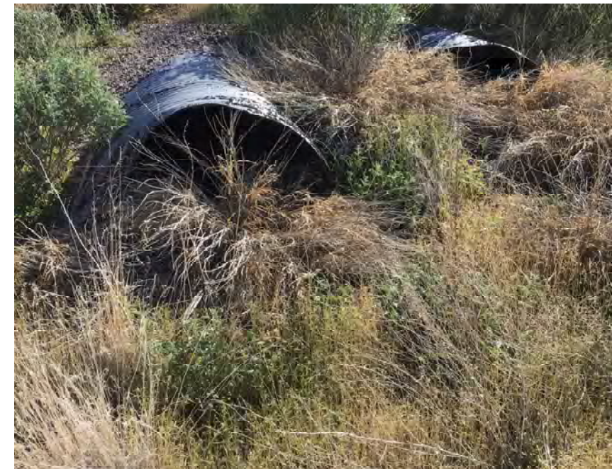
CULVERT #315 OUTLET (2) - 43" X 27" CMP ARCH STA 1297+00
