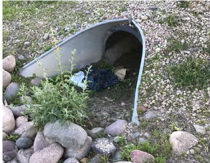
CULVERT #10 INLET 24" HDPE STA 929+00
