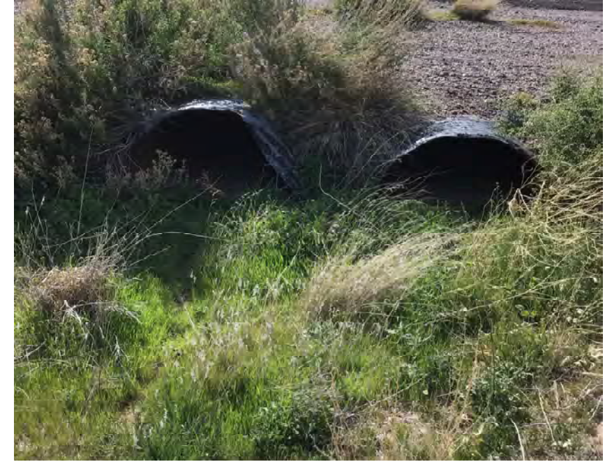
CULVERT #300 INLET (2) - 43" X 27" CMP ARCH STA 1285+00
