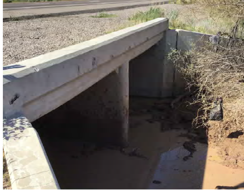
CULVERT #380 INLET BOX CULVERT 2-10' X 6' STA 1383+00
