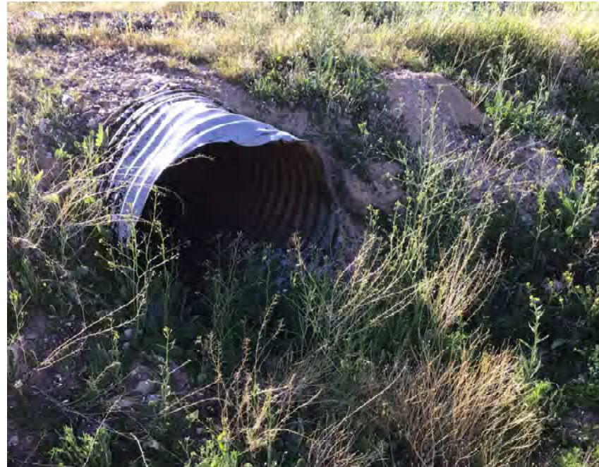
CULVERT #130 INLET 30" CMP STA 1093+00
