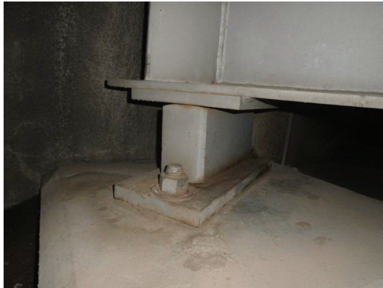
File Name : 01214-2020-05-31-Photo-12.JPG Description : Typical Bearing, N Abutment, LNW
