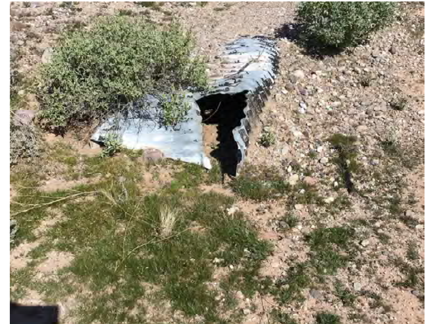
CULVERT #210 OUTLET 30" CMP STA 1201+50
