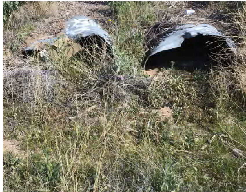
CULVERT #430 OUTLET (2) - 43" X 27" CMP ARCH STA 1448+00
