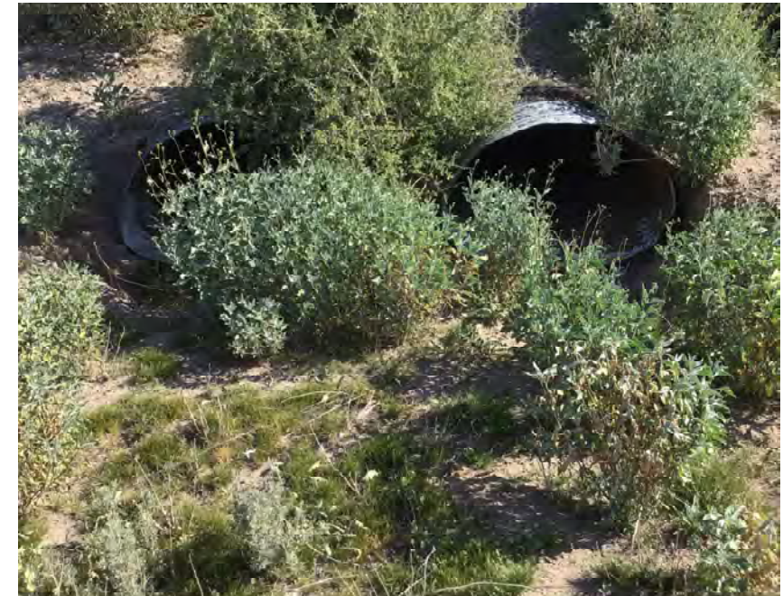
CULVERT #365 OUTLET (2) - 43" X 27" CMP ARCH STA 1359+00
