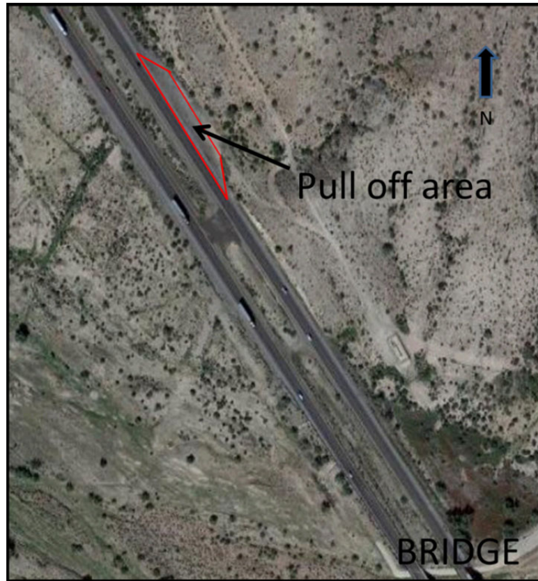
Figure 14: Pull off area
