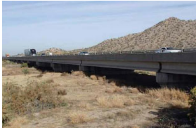
Figure 1: Bridge Elevation Looking North
