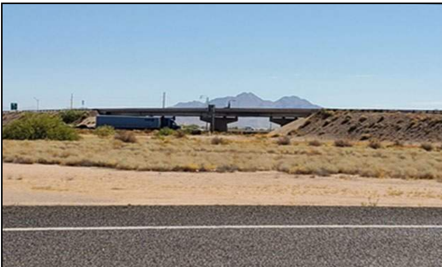
Figure 22. Typical view of a freeway bridge
