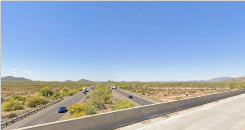
Figure 23. View north from State Route 387 overpass
