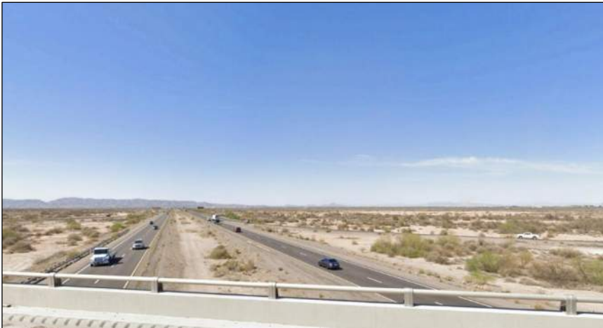
Figure 20. View north from Riggs Road overpass
