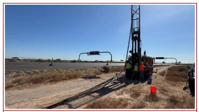
Photo 4: Typical layout for Ramps & Crossroads Boring
