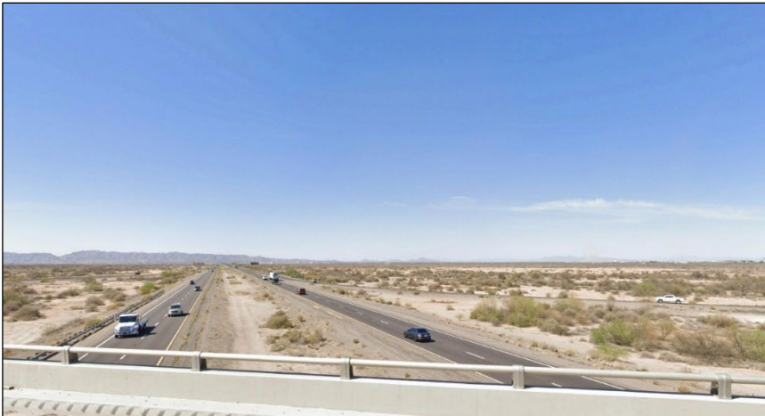
Figure 20. View north from Riggs Road overpass
