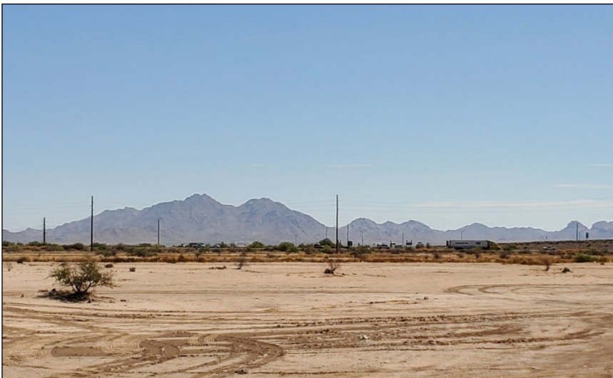
Figure 21. Typical view of the freeway main line
