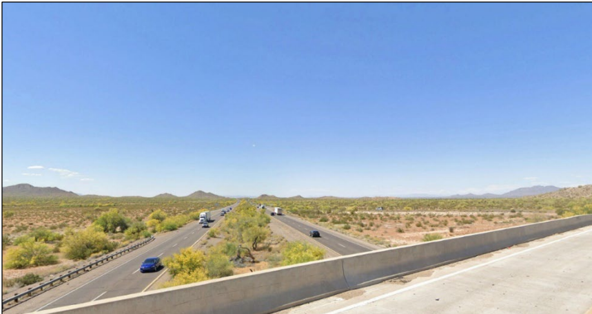
Figure 23. View north from State Route 387 overpass
