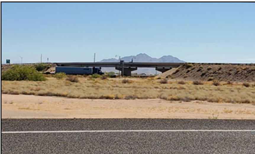
Figure 22. Typical view of a freeway bridge
