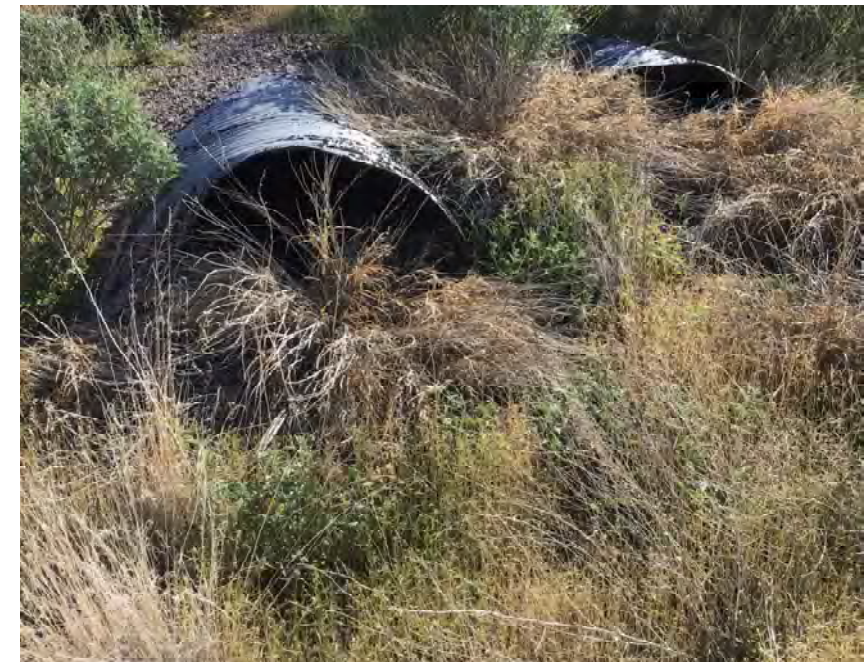
CULVERT #315 OUTLET (2) - 43" X 27" CMP ARCH STA 1297+00
