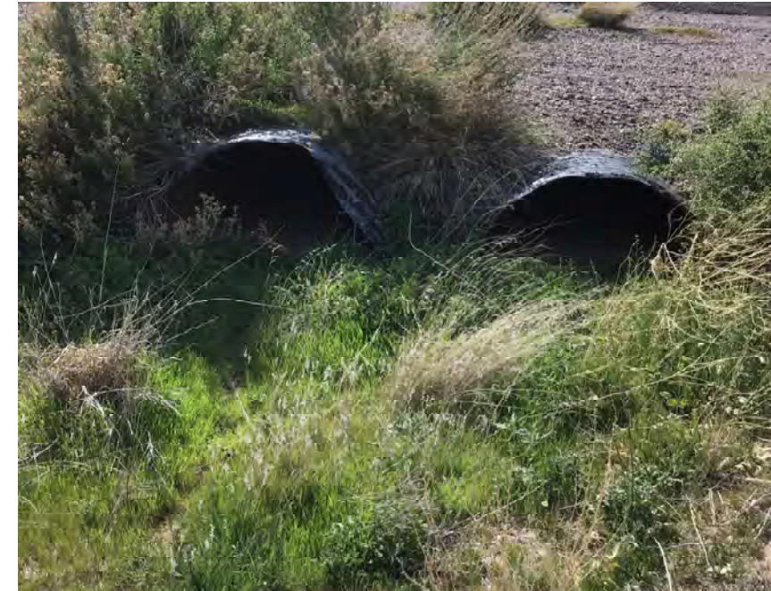
CULVERT #300 INLET (2) - 43" X 27" CMP ARCH STA 1285+00
