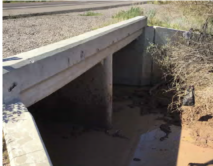
CULVERT #380 INLET BOX CULVERT 2-10' X 6' STA 1383+00
