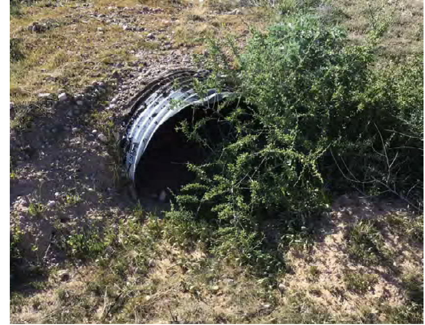
CULVERT #175 INLET 36" X 22" CMP ARCH STA 1136+50
