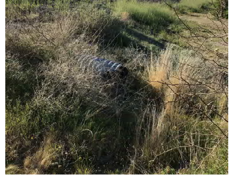
CULVERT #125 INLET 30" CMP STA 1083+00
