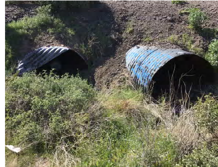
CULVERT #435 INLET (2) - 58" X 36" CMP ARCH STA 1461+83
