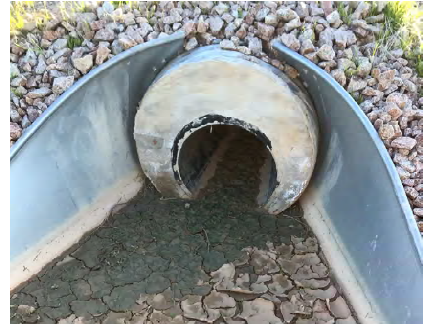
CULVERT #65 INLET 18" CMP STA 1008+10
