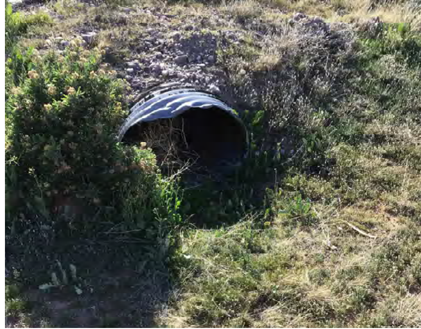
CULVERT #150 INLET 29" X 18" CMP ARCH STA 1117+00
