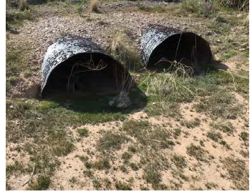
CULVERT #280 INLET (2) - 43" X 27" CMP ARCH STA 1261+00
