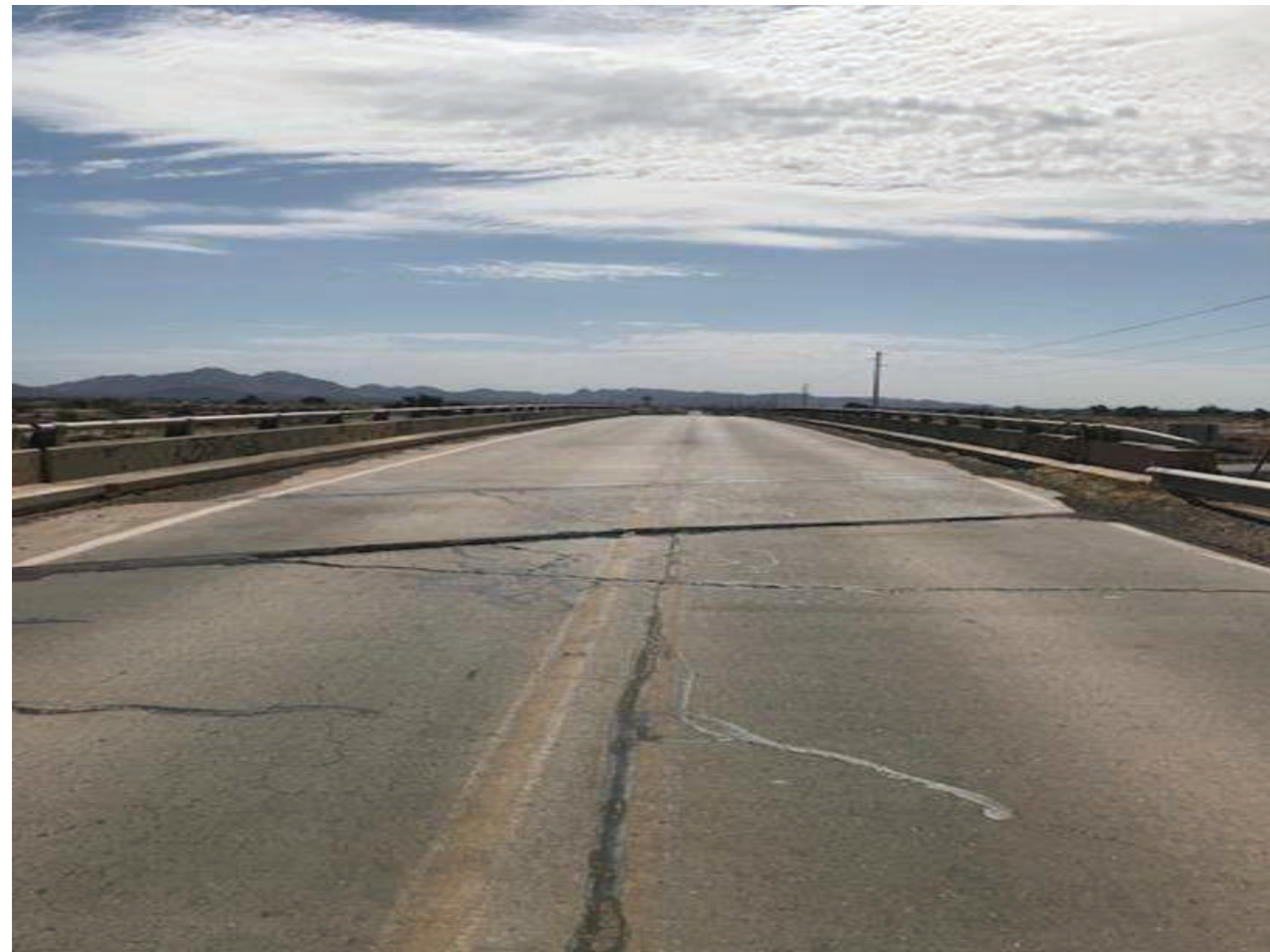
File Name : 01213-2021-05-18-Photo-1.jpg Description : Roadway ID looking E
