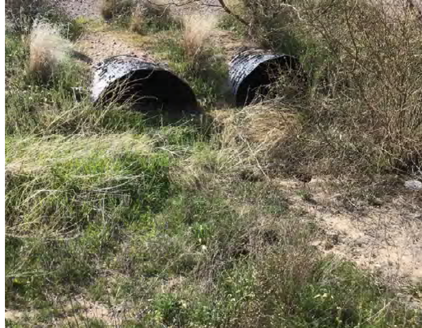
CULVERT #285 INLET (2) - 43" X 27" CMP ARCH STA 1267+00
