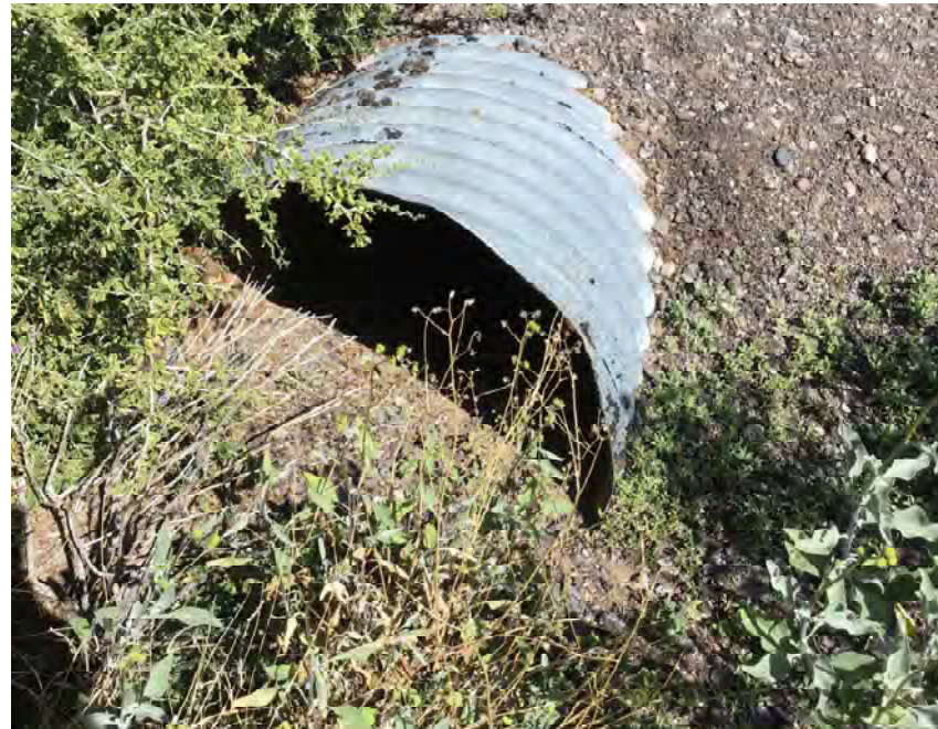
CULVERT #205 OUTLET 30" CMP STA 1198+50
