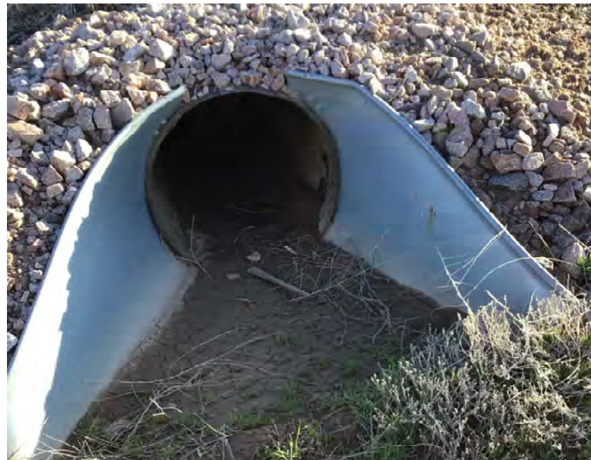
CULVERT #60 OUTLET 30" CMP STA 1002+50
