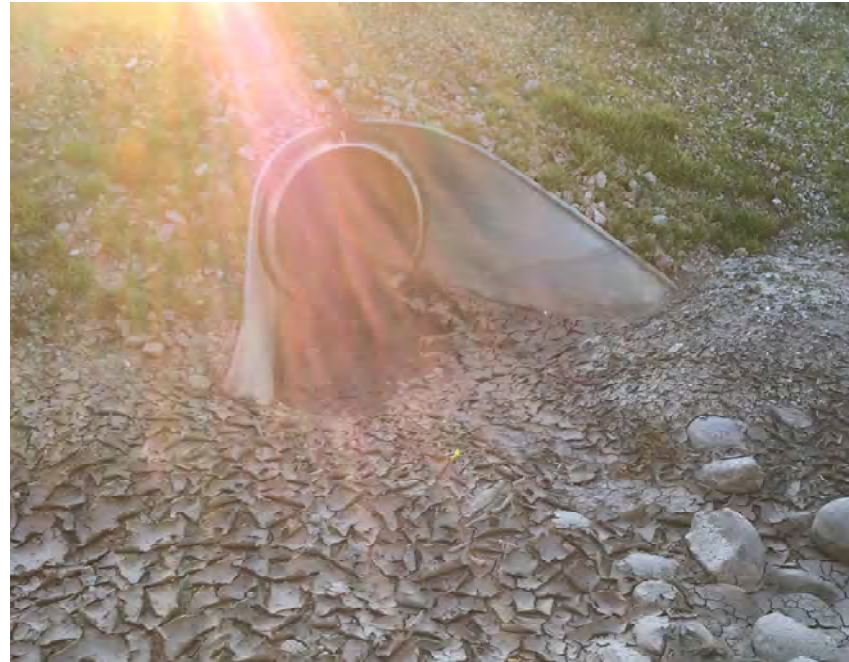
CULVERT #20 INLET 30" HDPE STA 945+10
