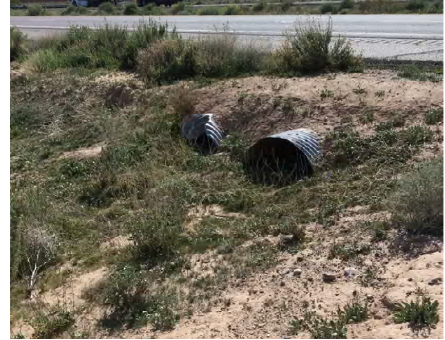
CULVERT #315 INLET (2) - 43" X 27" CMP ARCH STA 1297+00
