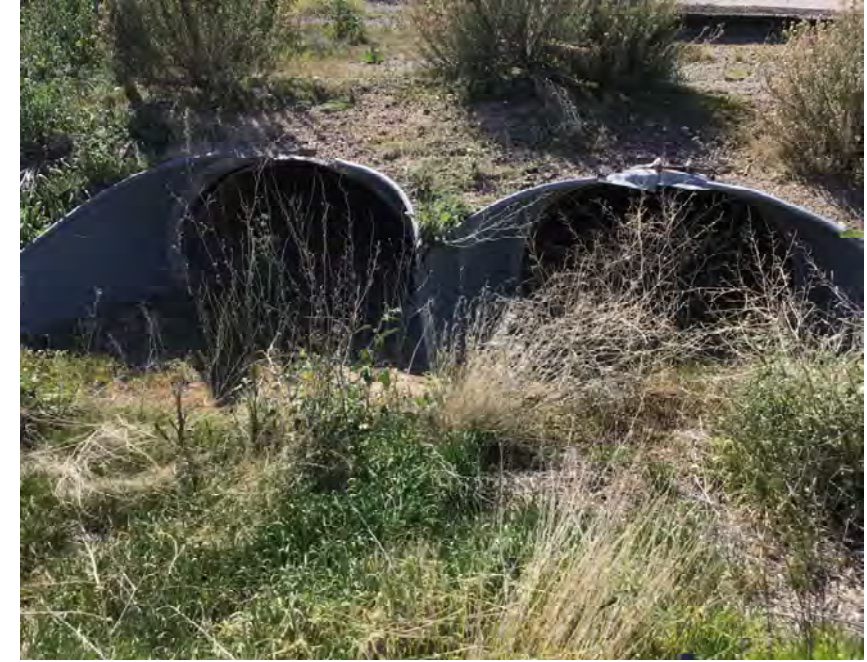
CULVERT #335 INLET (2) - 43" X 27" CMP ARCH STA 1323+00
