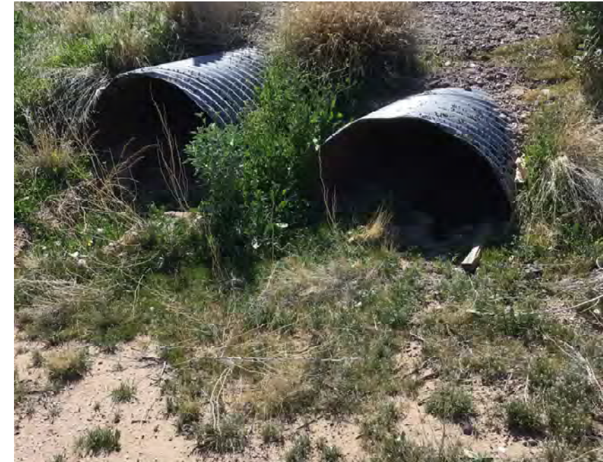
CULVERT #365 INLET (2) - 43" X 27" CMP ARCH STA 1359+00
