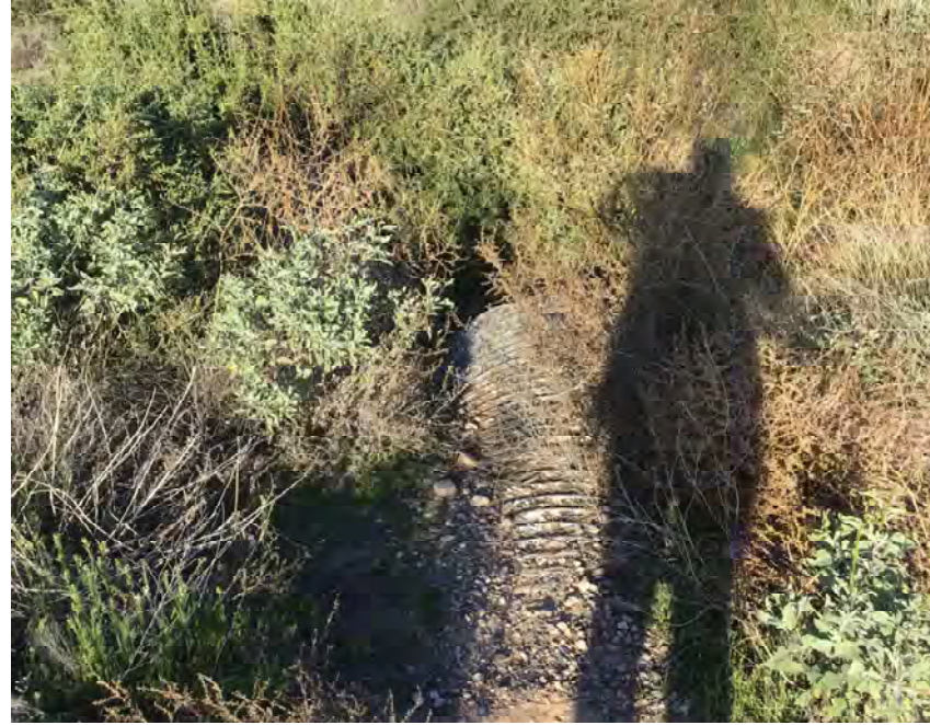
CULVERT #80 INLET 36" X 22" CMP ARCH STA 1029+00
