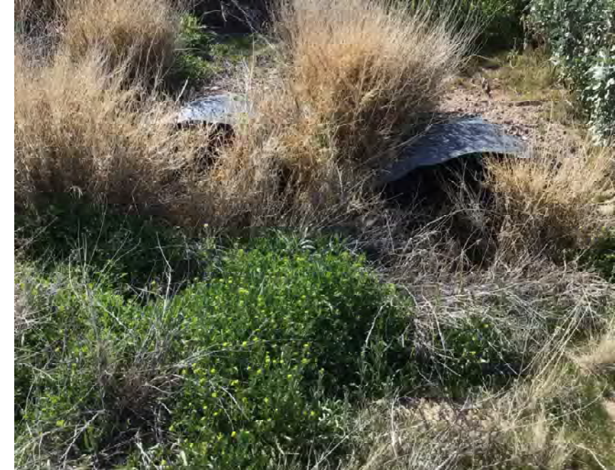
CULVERT #405 INLET (2) - 43" X 27" CMP ARCH STA 1417+00
