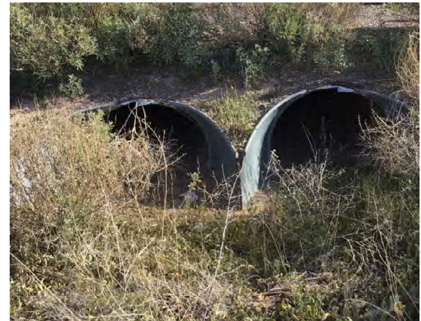
CULVERT #335 OUTLET (2) - 43" X 27" CMP ARCH STA 1323+00
