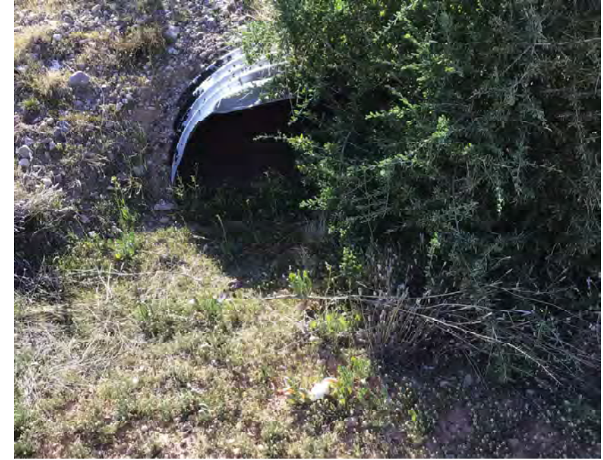
CULVERT #155 INLET 29" X 18" CMP ARCH STA 1124+50
