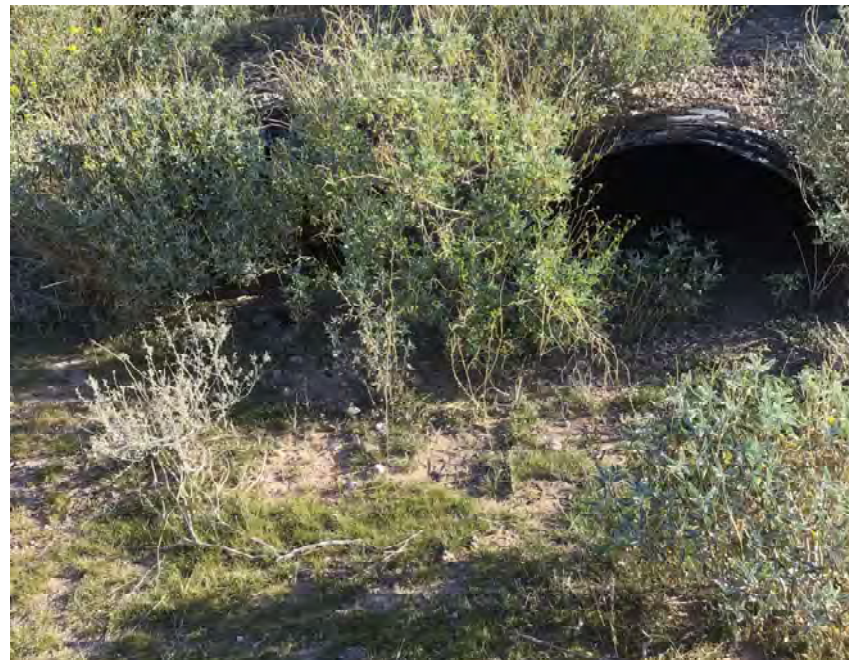
CULVERT #285 OUTLET (2) - 43" X 27" CMP ARCH STA 1267+00
