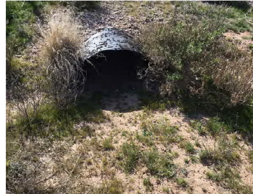
CULVERT #240 INLET 36" X 22" CMP ARCH STA 1233+00
