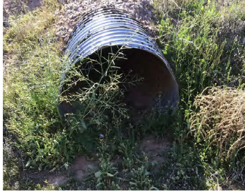
CULVERT #140 INLET 30" CMP STA 1105+50
