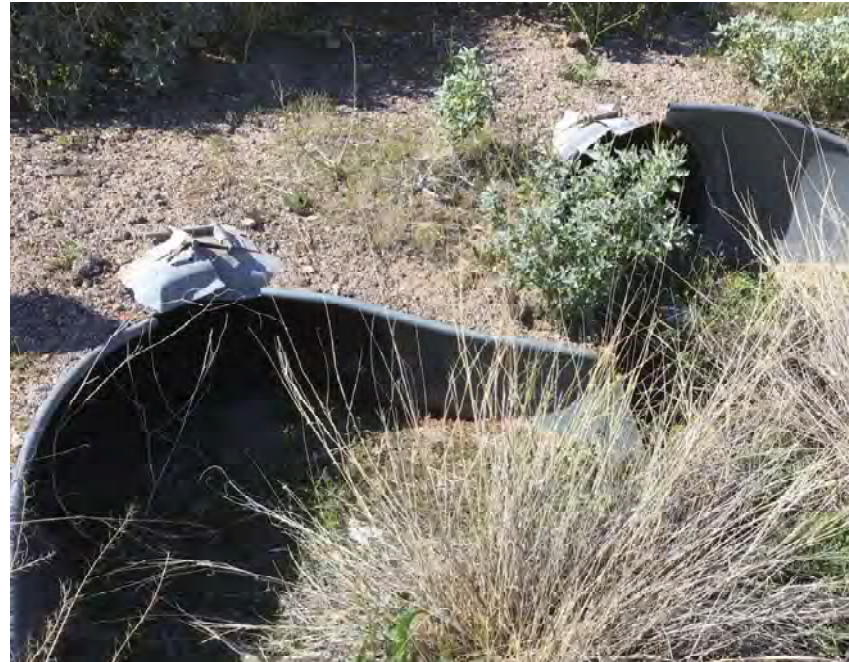
CULVERT #430 INLET (2) - 43" X 27" CMP ARCH STA 1448+00
