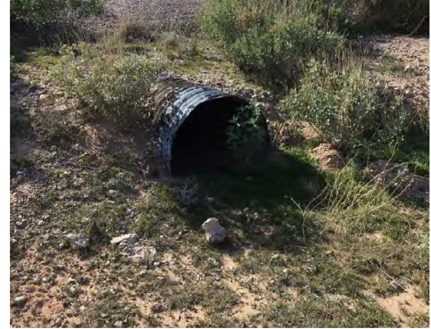
CULVERT #210 INLET 30" CMP STA 1201+50
