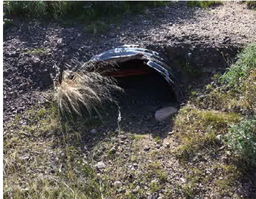
CULVERT #235 INLET 36" X 22" CMP ARCH STA 1224+00
