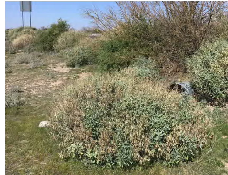
CULVERT #230 OUTLET 36" X 22" CMP ARCH STA 1220+00
