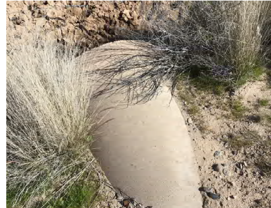
CULVERT #385 INLET 30" RCP STA 1385+44
