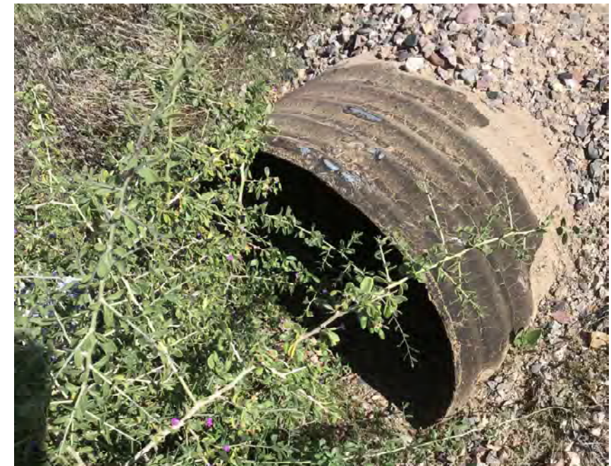
CULVERT #155 OUTLET 29" X 18" CMP ARCH STA 1124+50
