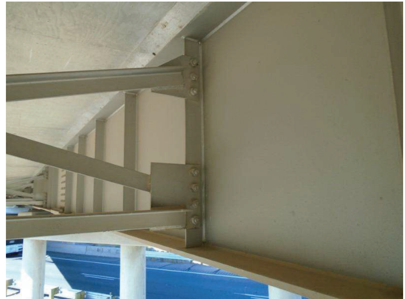
File Name : 01215-2020-05-31-Photo-17.JPG Description : Typical Diaphragm Connection
