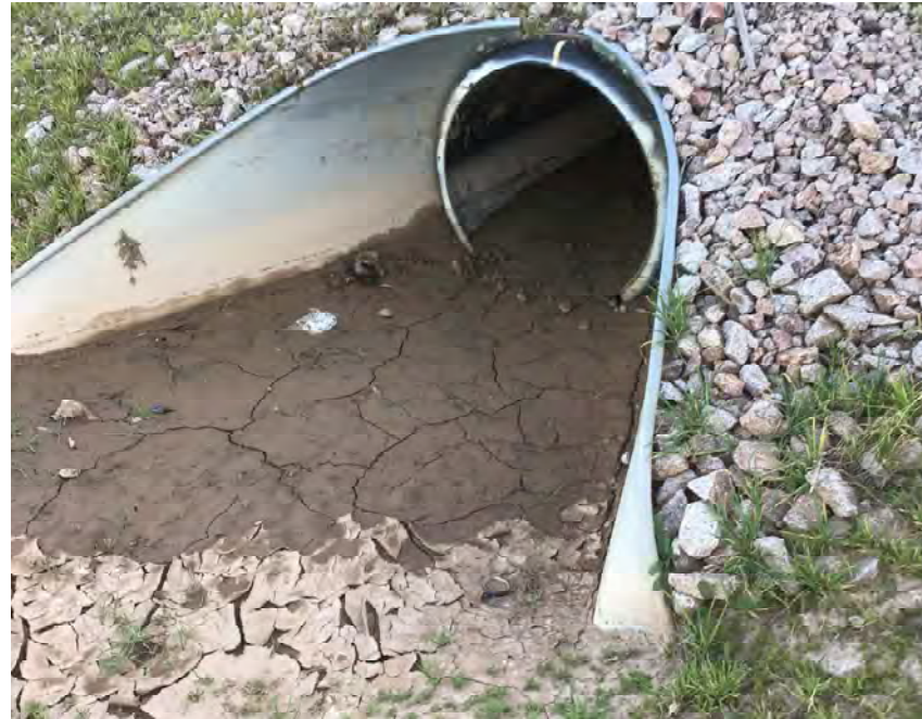
CULVERT #30 INLET 30" HDPE STA 954+25
