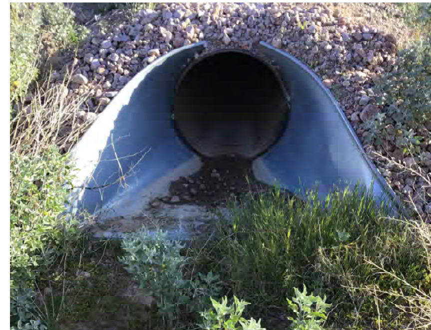
CULVERT #75 OUTLET 30" CMP STA 1018+00
