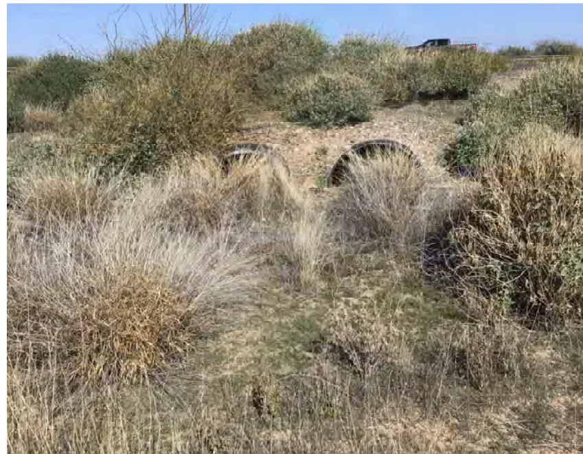
CULVERT #275 OUTLET (2) 43" X 27" CMP ARCH STA 1255+00
