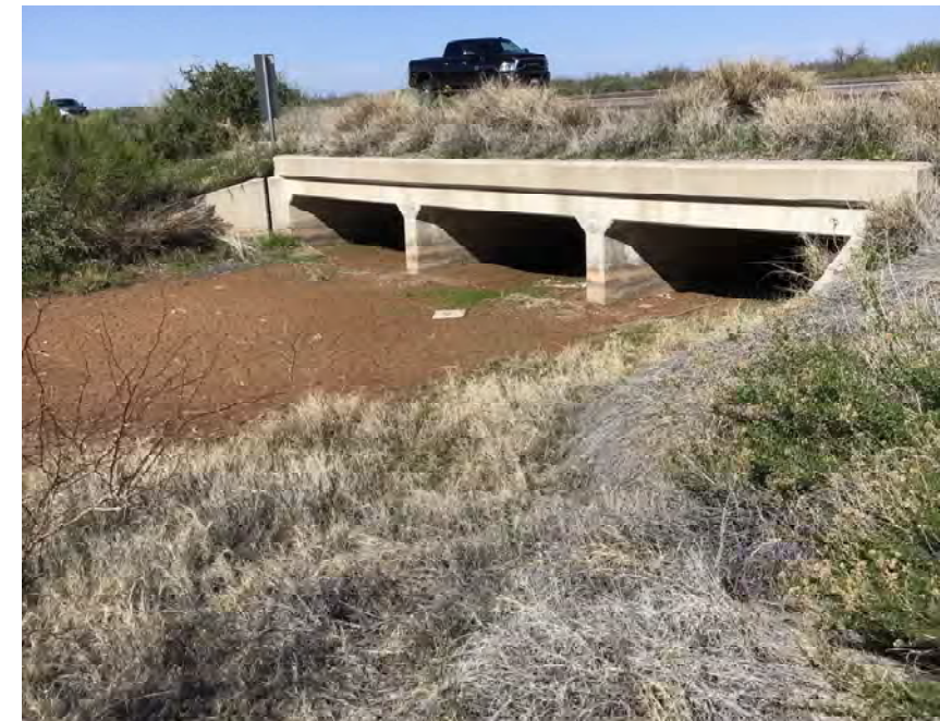
CULVERT #250 OUTLET BOX CULVERT 3- 10' X 3' STA 1240+33
