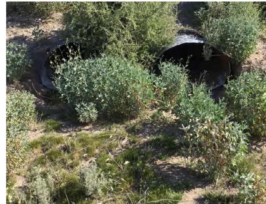
CULVERT #365 OUTLET (2) - 43" X 27" CMP ARCH STA 1359+00
