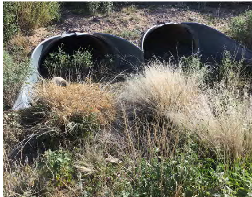
CULVERT #330 OUTLET (2) - 43" X 27" CMP ARCH STA 1317+00
