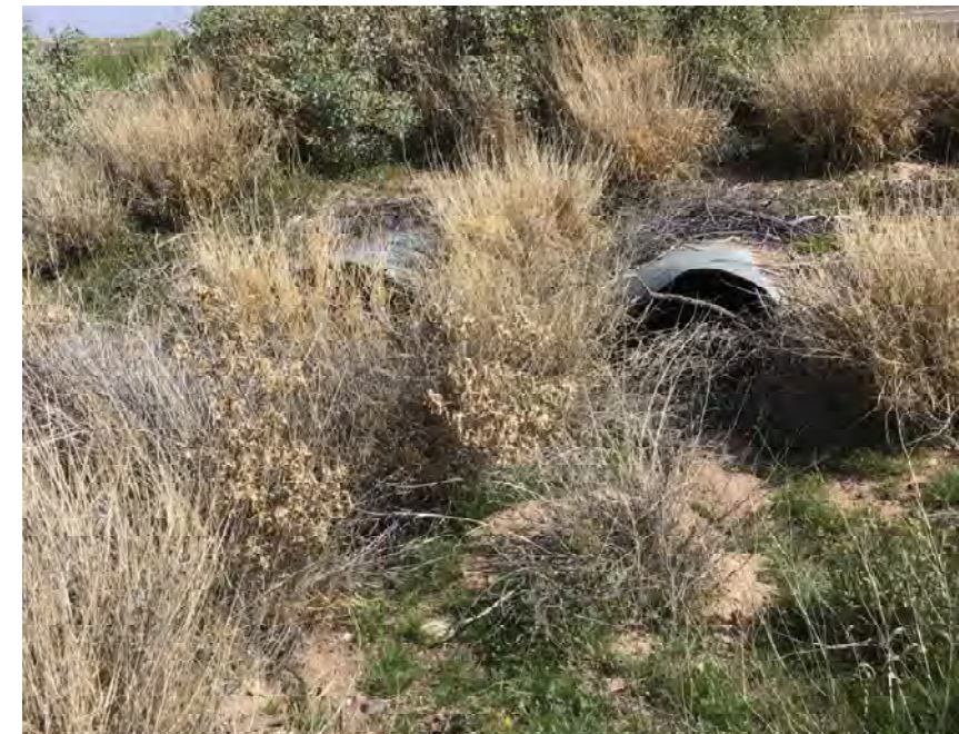
CULVERT #405 OUTLET (2) - 43" X 27" CMP ARCH STA 1417+00
