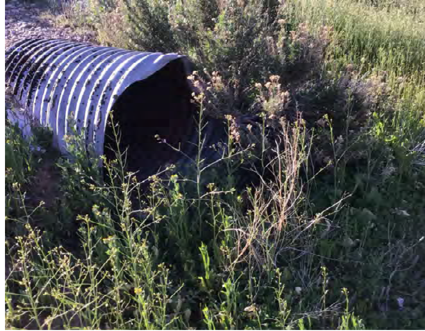
CULVERT #120 INLET 30" CMP STA 1077+00
