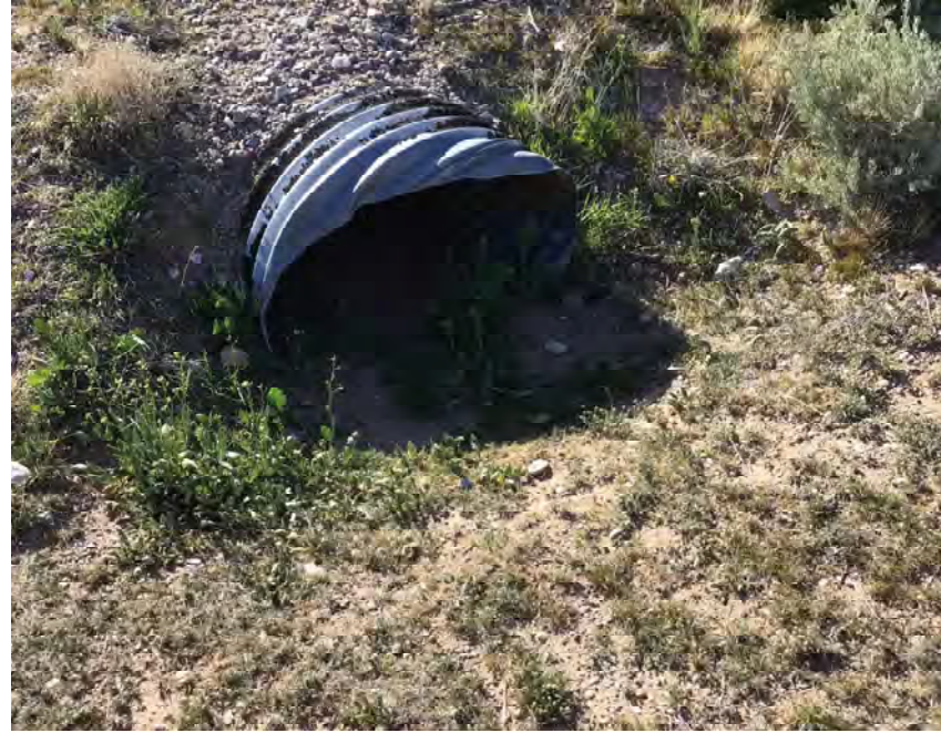
CULVERT #170 INLET 29" X 18" STA 1133+50
