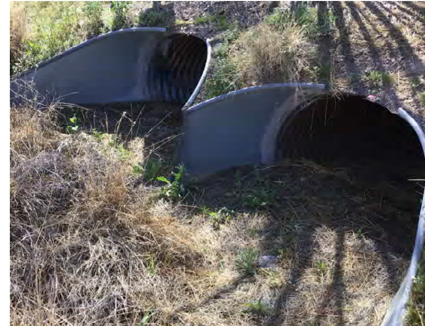
CULVERT #425 INLET (2) - 43" X 27" CMP ARCH STA 1442+00
