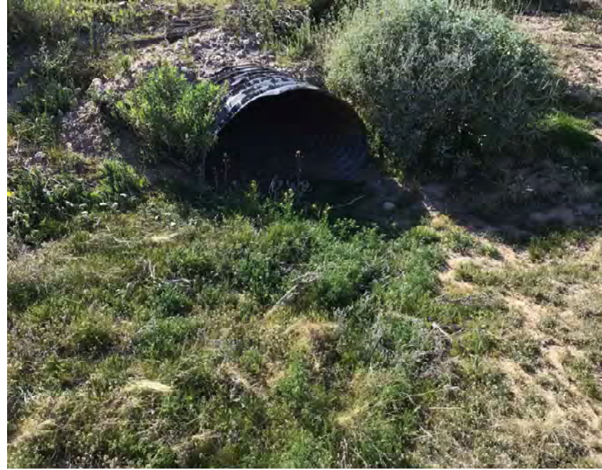
CULVERT #180 INLET 36" X 22" CMP ARCH STA 1143+50
