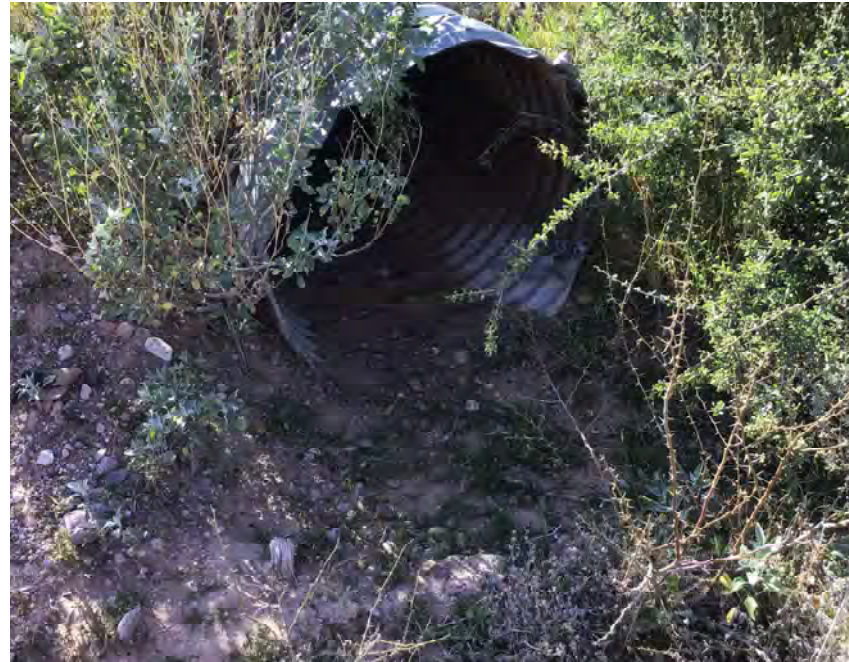
CULVERT #190 INLET 30" CMP STA 1156+56
