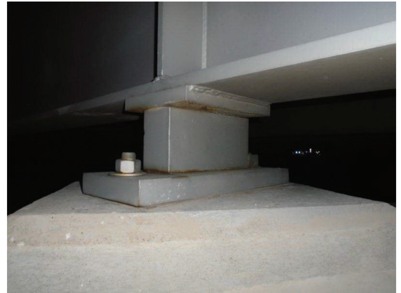
File Name : 01214-2020-05-31-Photo-17.JPG Description : Typical Bearing, Pier 3, LS
