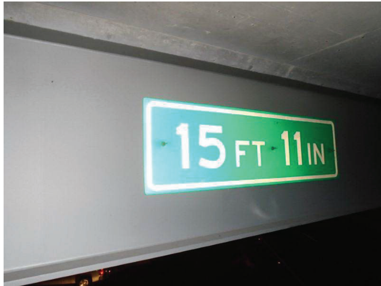
File Name : 01214-2020-05-31-Photo-30.JPG Description : EB Clearance Sign, 15'-11", LE
