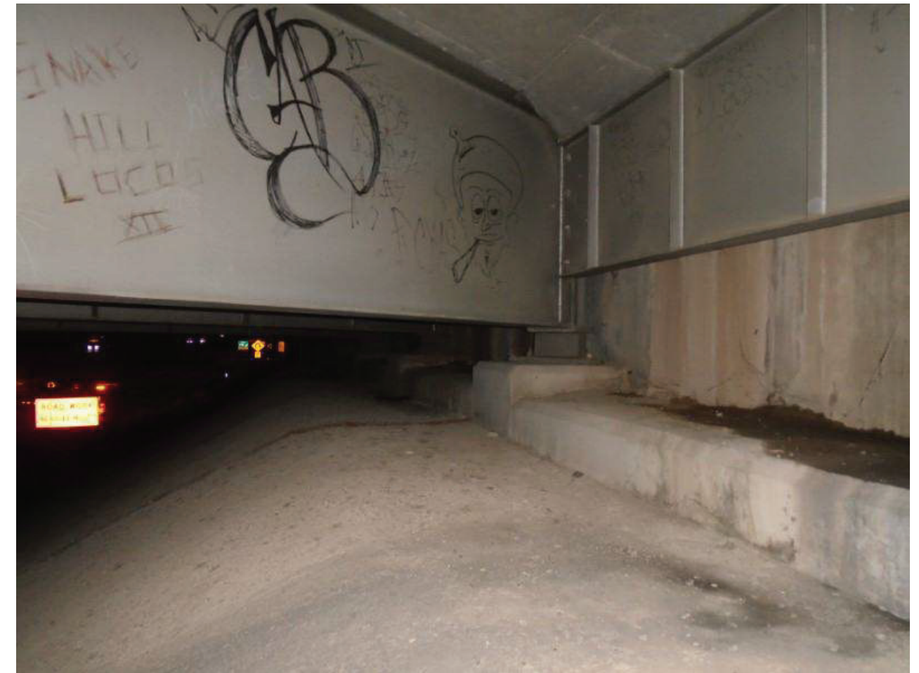
File Name : 01214-2020-05-31-Photo-19.JPG Description : South Abutment, LSE
