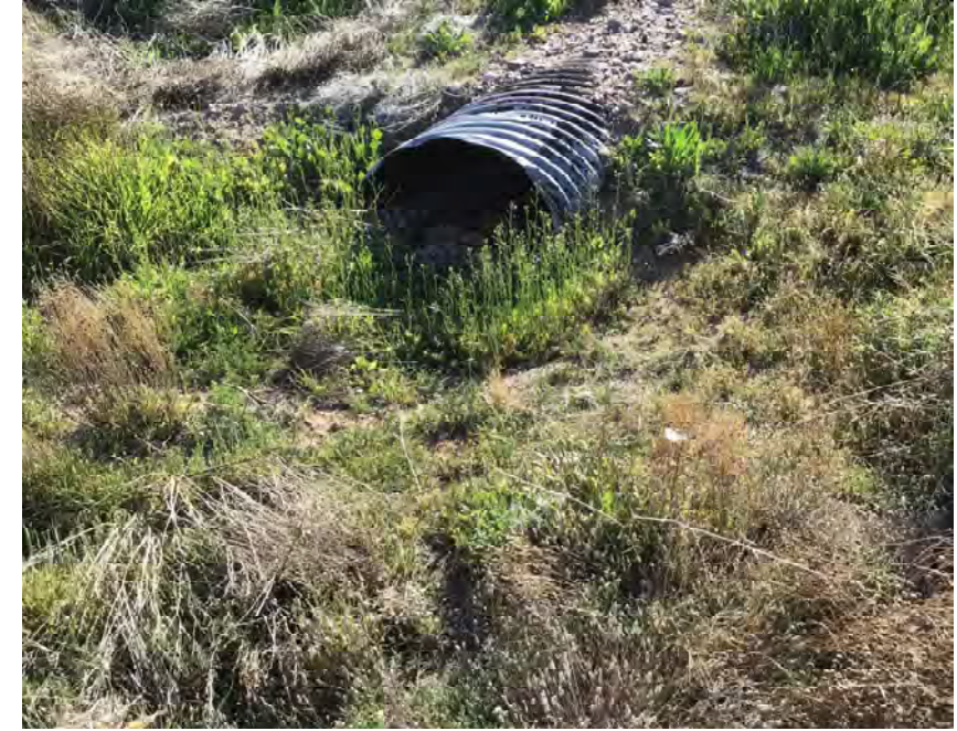
CULVERT #165 INLET 29" X 18" CMP ARCH STA 1130+00
