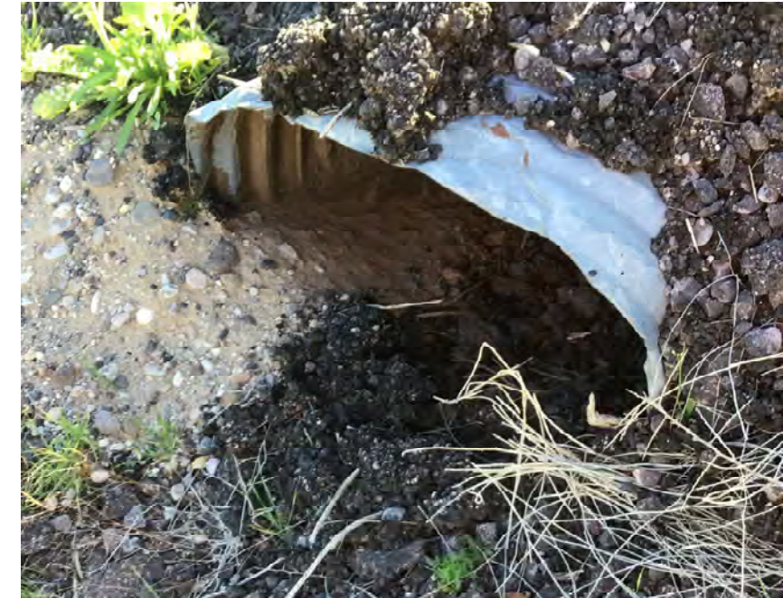
CULVERT #135 INLET 30" CMP STA 1097+00
