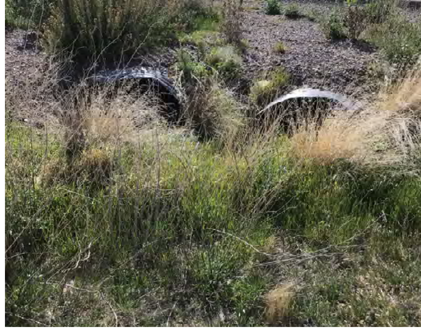
CULVERT #330 INLET (2) - 43" X 27" CMP ARCH STA 1317+00
