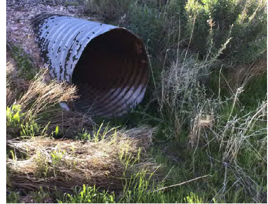
CULVERT #105 INLET 30" CMP STA 1061+00
