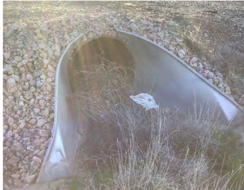
CULVERT #60 INLET 30" CMP STA 1002+50
