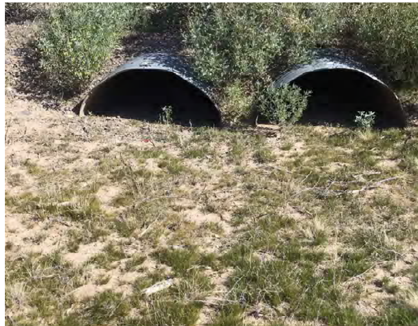
CULVERT #420 OUTLET (2) - 43" X 27" CMP ARCH STA 1435+00
