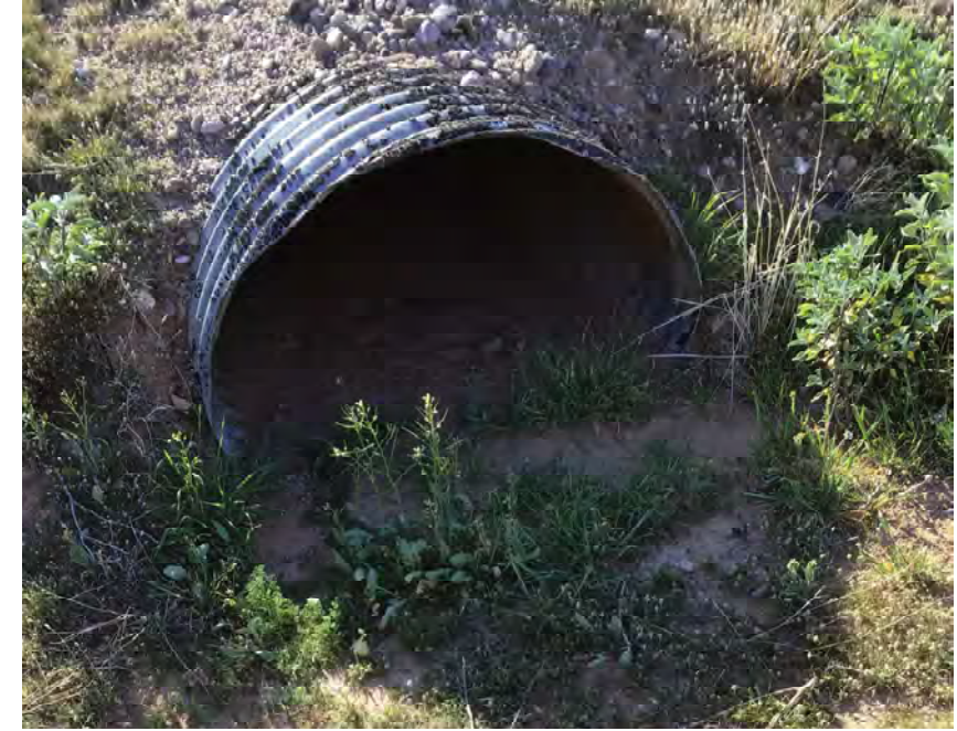
CULVERT #145 INLET 36" X 22" CMP ARCH STA 1109+00
