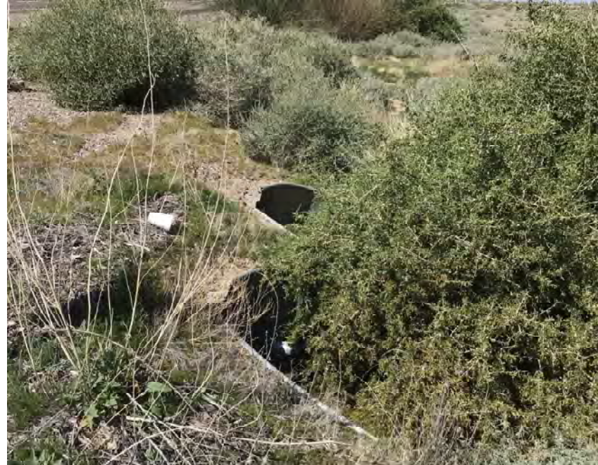
CULVERT #390 INLET (3) - 43" X 27" CMP ARCH STA 1395+00
