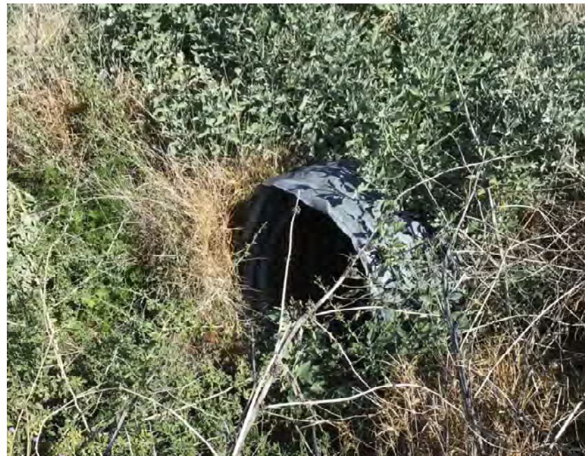
CULVERT #100 OUTLET 36" X 22" CMP ARCH STA 1050+00
