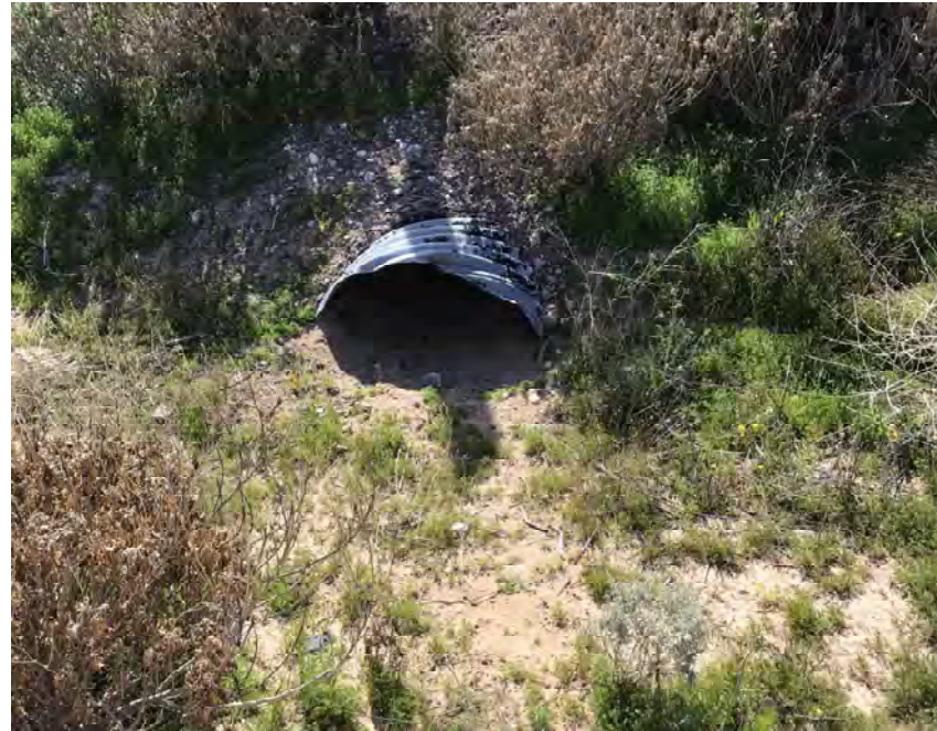
CULVERT #245 INLET 29" X 18" CMP ARCH STA 1237+00
