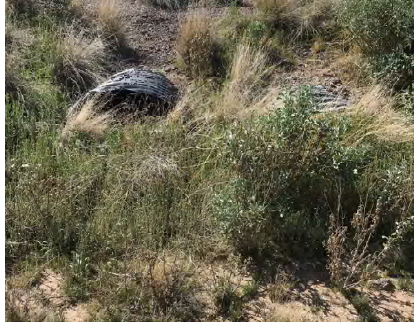
CULVERT #410 INLET (2) - 43" X 27" CMP ARCH STA 1423+00
