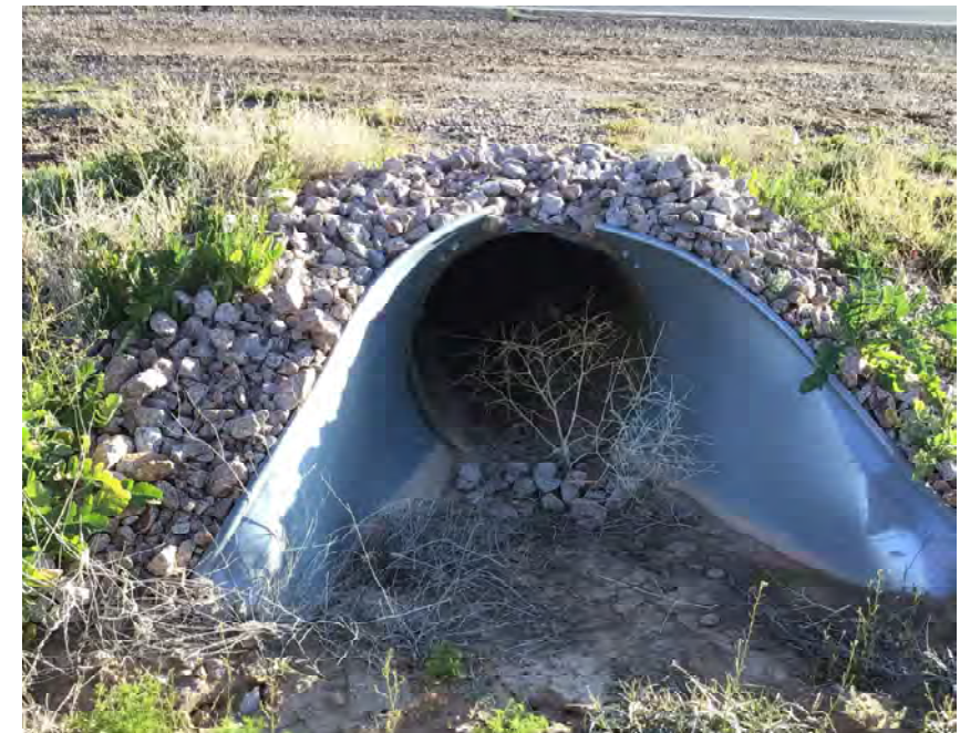
CULVERT #65 OUTLET 30" CMP STA 1008+10
