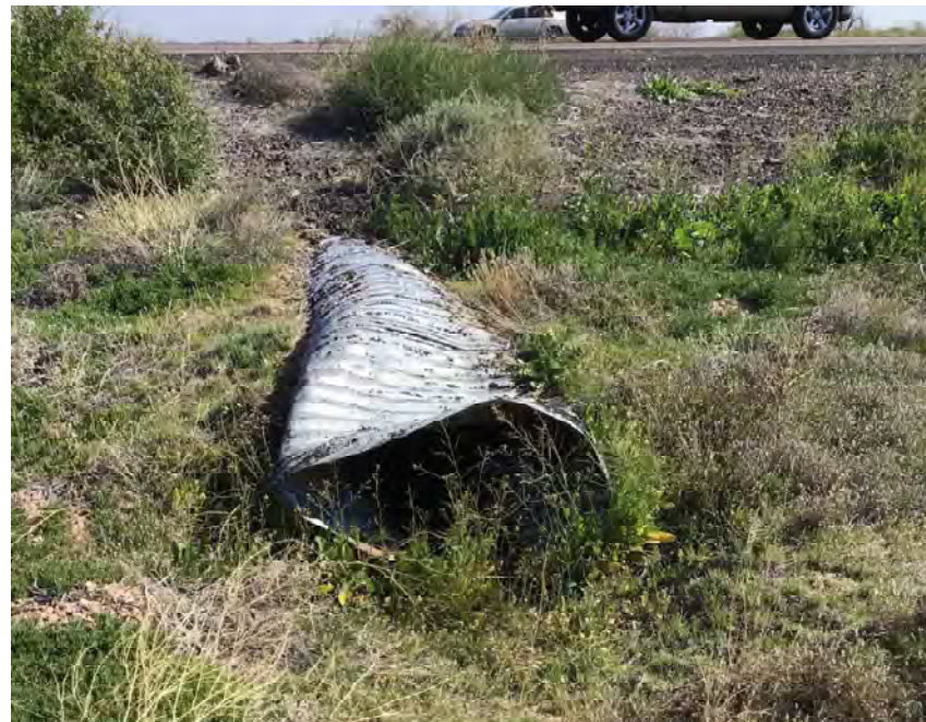
CULVERT #120 OUTLET 30" CMP STA 1077+00
