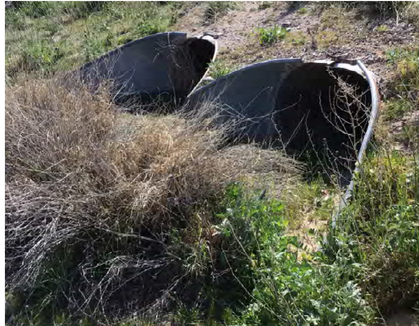
CULVERT #350 INLET (2) - 43" X 27" CMP ARCH STA 1341+00
