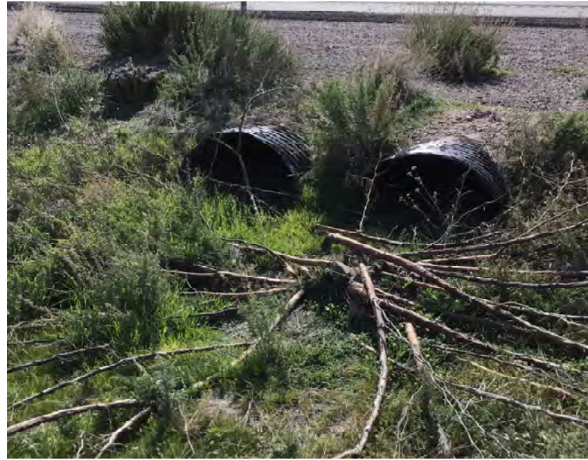
CULVERT #255 INLET (2) - 43" X 27" CMP ARCH STA 1243+00
