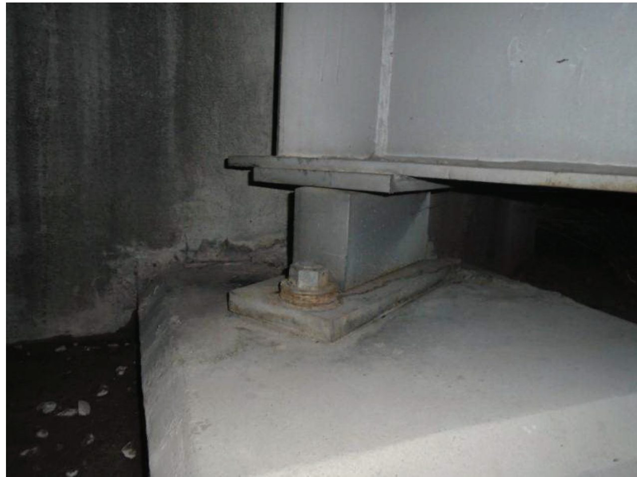
File Name : 01214-2020-05-31-Photo-18.JPG Description : Typical Bearing, S Abutment, LNw
