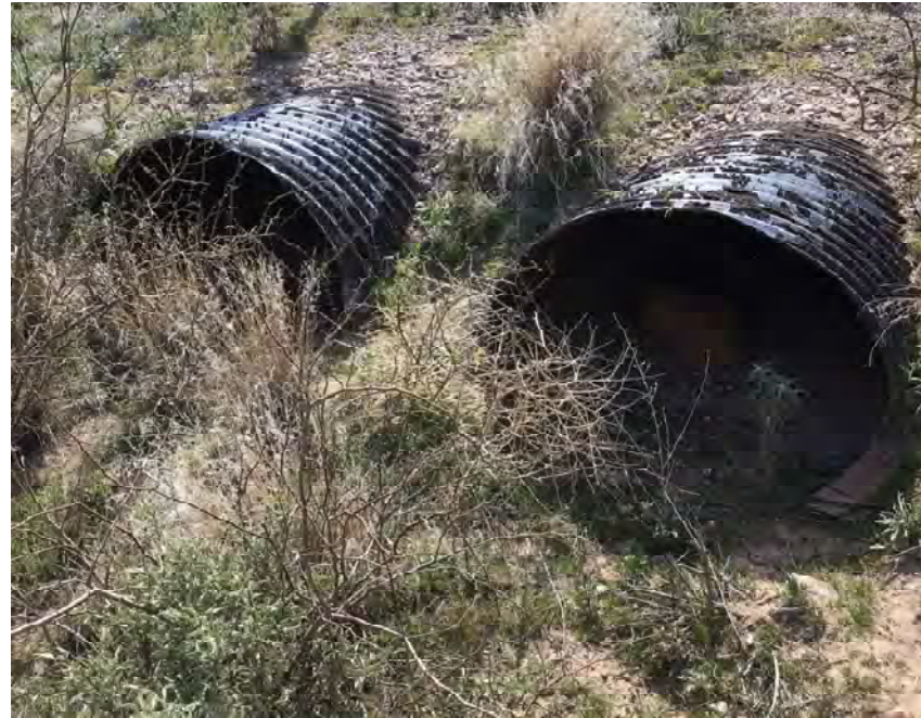
CULVERT #295 INLET (2) - 43" X 27" CMP ARCH STA 1279+00
