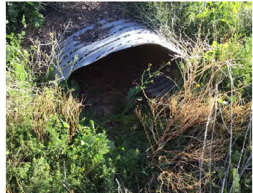
CULVERT #95 OUTLET 36" X 22" CMP ARCH STA 1047+00
