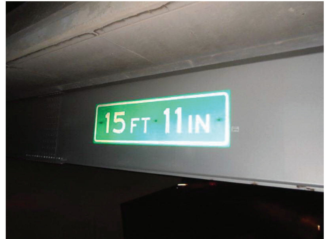
File Name : 01214-2020-05-31-Photo-29.JPG Description : WB Clearance Sign, 15'-11", LNW
