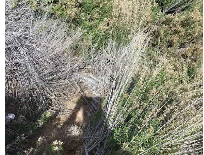
CULVERT #290 INLET (2) - 43" X 27" CMP ARCH STA 1273+00
