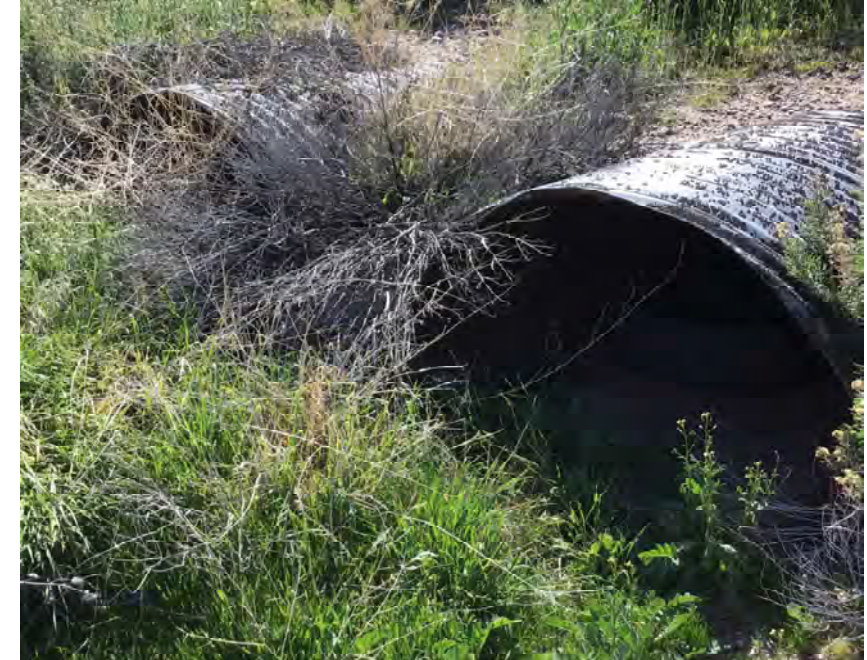
CULVERT #375 INLET (2) - 58" X 36" CMP ARCH STA 1378+00
