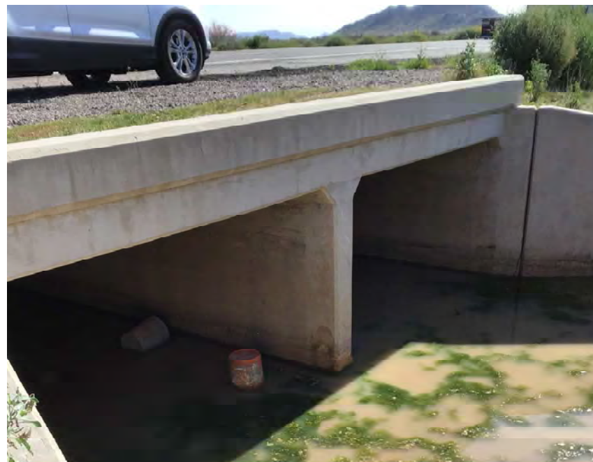
CULVERT #380 OUTLET BOX CULVERT 2-10' X 6' STA 1383+00
