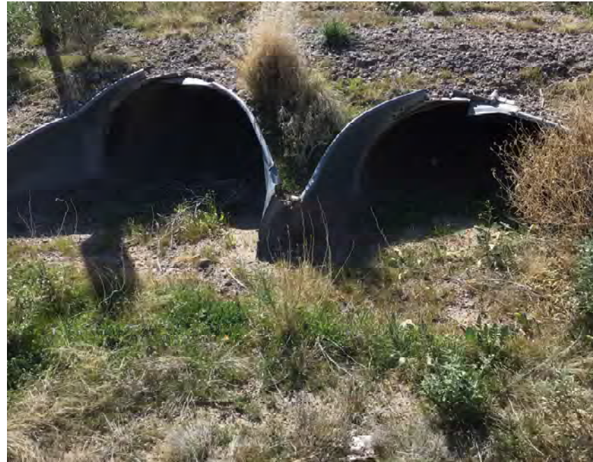
CULVERT #360 INLET (2) - 43" X 27" CMP ARCH STA 1353+00
