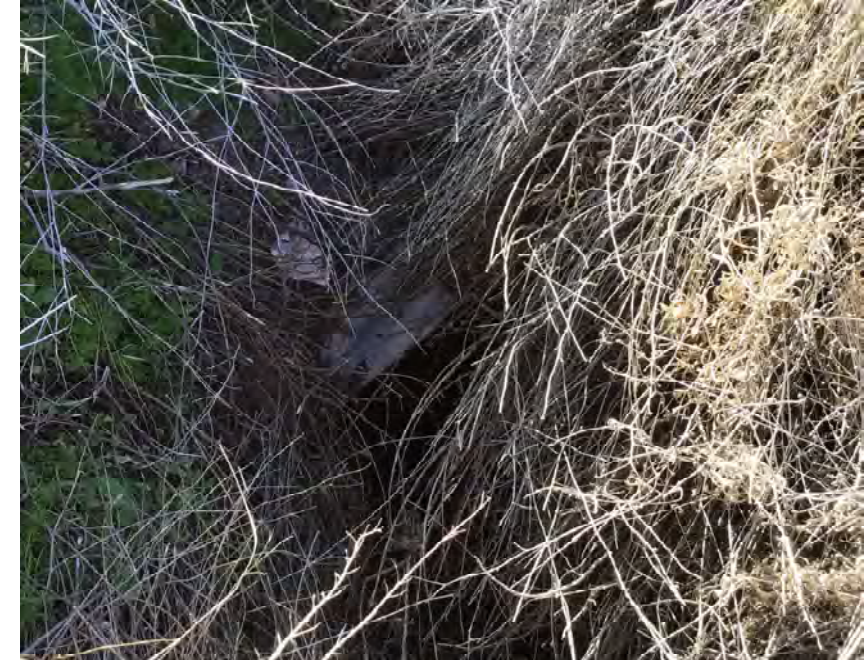
CULVERT #95 INLET 36" X 22" CMP ARCH STA 1047+00
