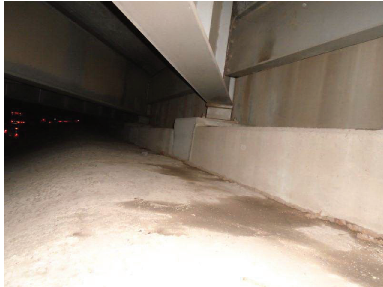
File Name : 01215-2020-05-31-Photo-16.JPG Description : South Abutment, LSE
