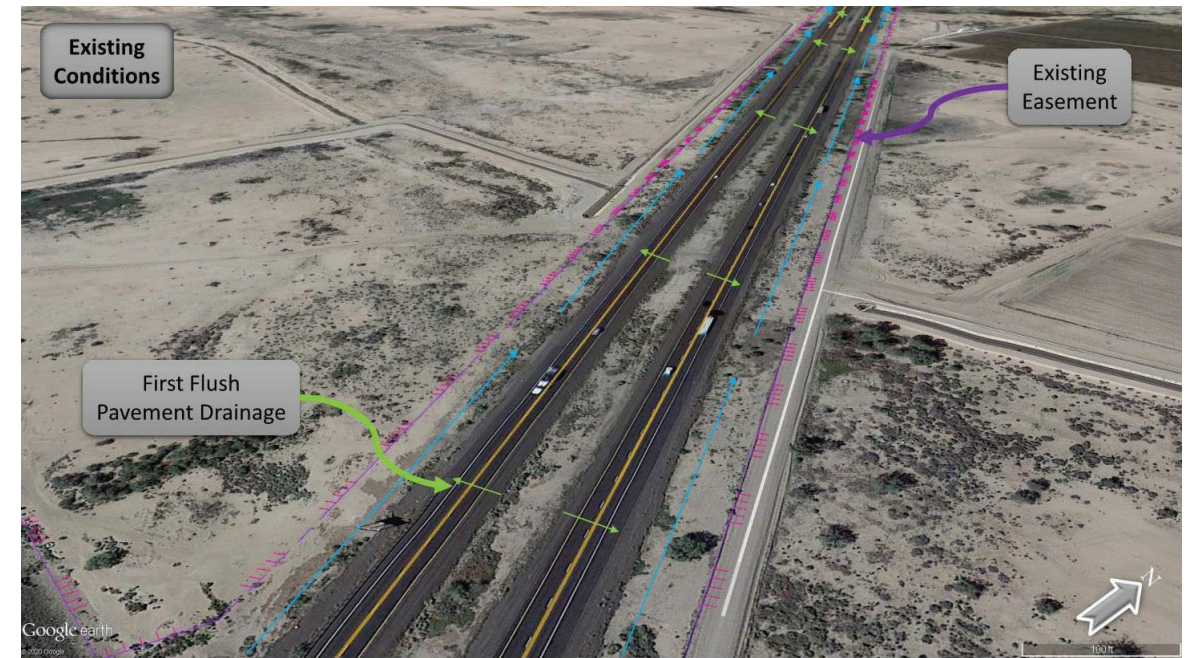
Exhibit 2a: Gila River to SR-587 – Existing Condition
