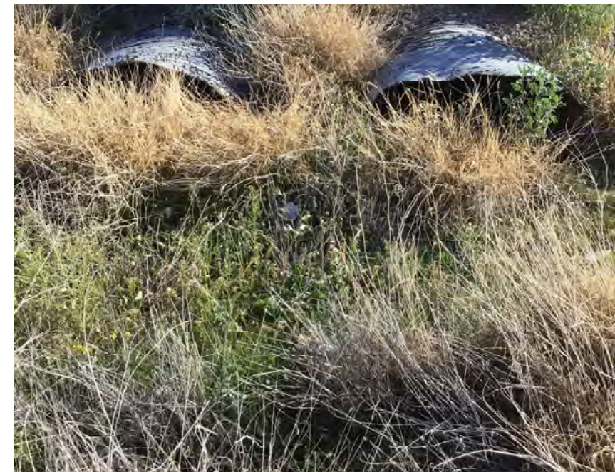
CULVERT #300 OUTLET (2) - 43" X 27" CMP ARCH STA 1285+00
