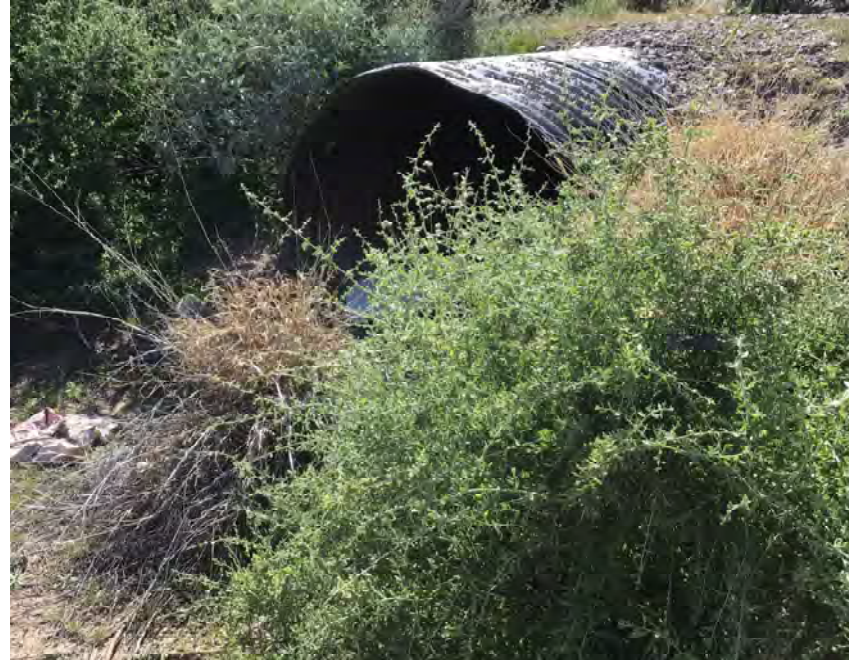
CULVERT #370 INLET (2) - 58" X 36" CMP ARCH STA 1371+00
