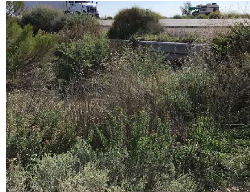
CULVERT #250 INLET BOX CULVERT 3- 10' X 3' STA 1240+33
