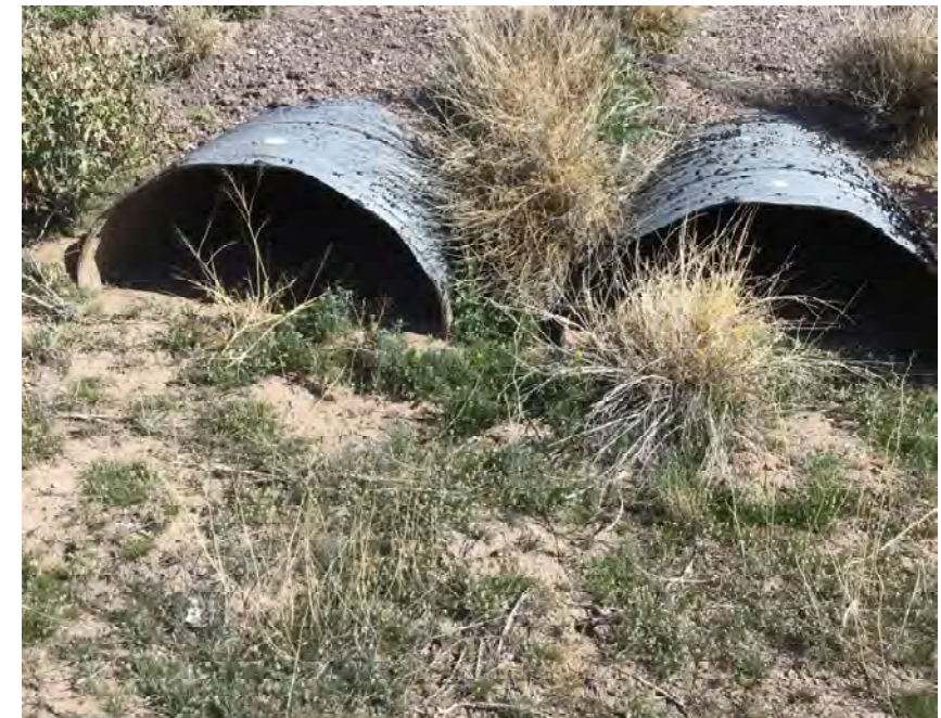
CULVERT #415 OUTLET (2) - 43" X 27" CMP ARCH STA 1429+00
