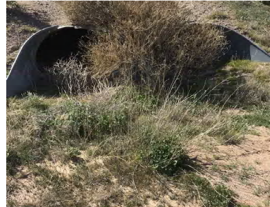
CULVERT #325 INLET (2) - 43" X 27" CMP ARCH STA 1311+00
