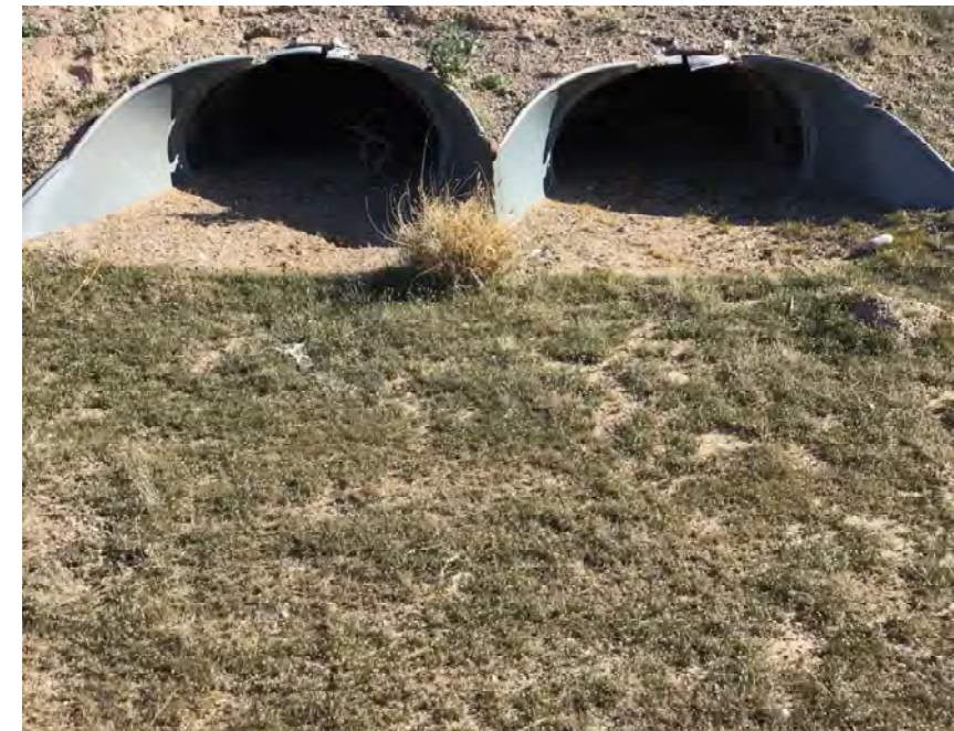
CULVERT #355 OUTLET (2) - 43" X 27" CMP ARCH STA 1347+00
