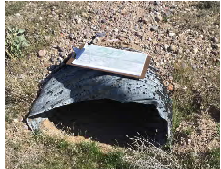
CULVERT #145 OUTLET 36" X 22" CMP ARCH STA 1109+00
