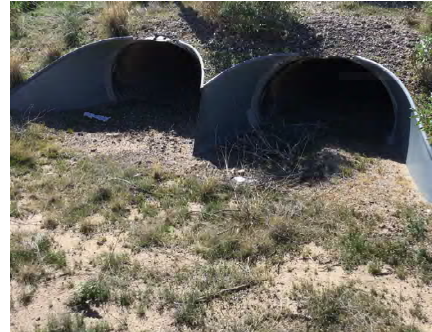
CULVERT #355 INLET (2) - 43" X 27" CMP ARCH STA 1347+00
