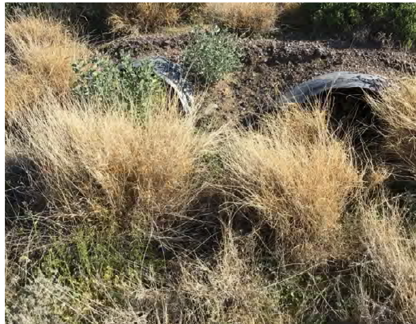
CULVERT #360 OUTLET (2) - 43" X 27" CMP ARCH STA 1353+00
