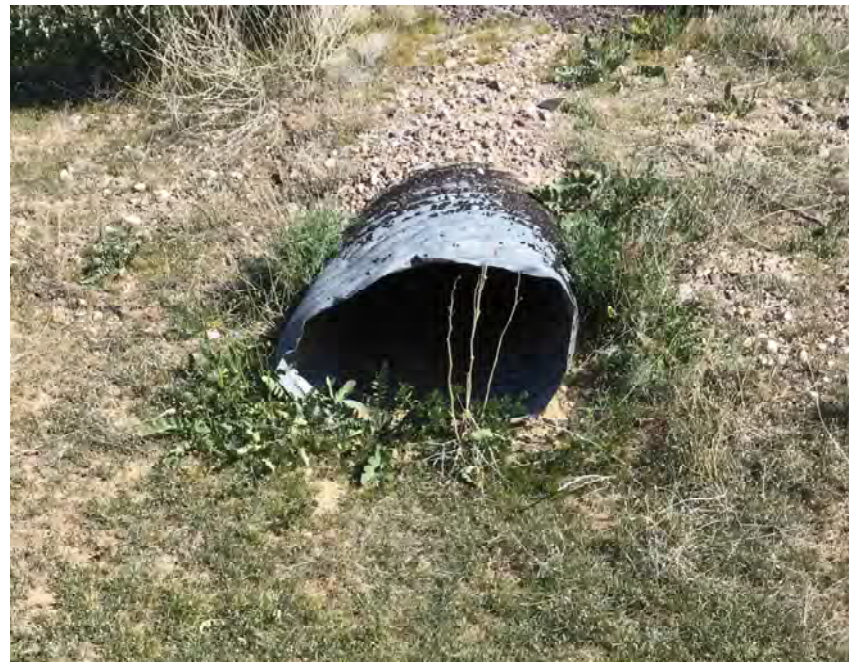
CULVERT #170 OUTLET 29" X 18" STA 1133+50
