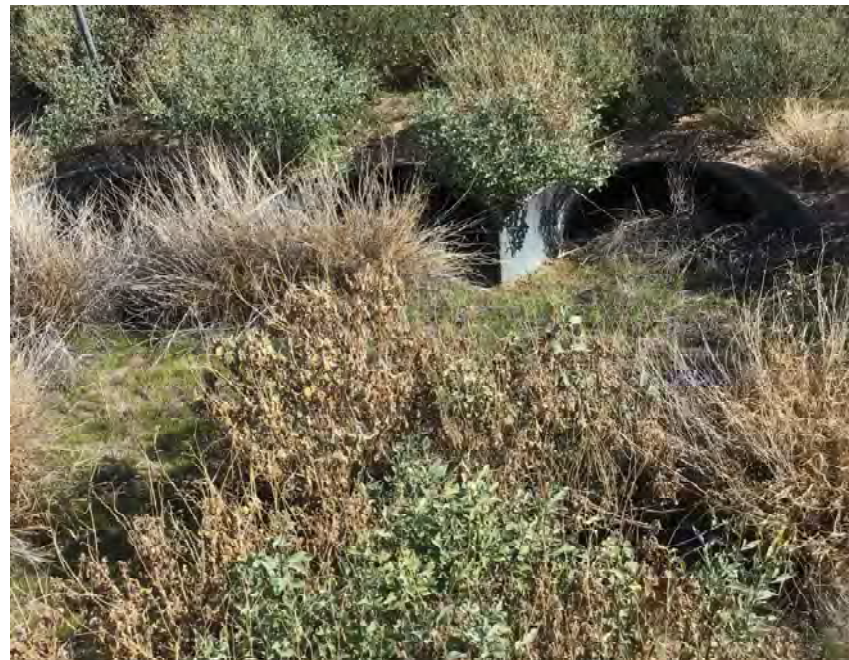
CULVERT #390 OUTLET (3) - 43" X 27" CMP ARCH STA 1395+00
