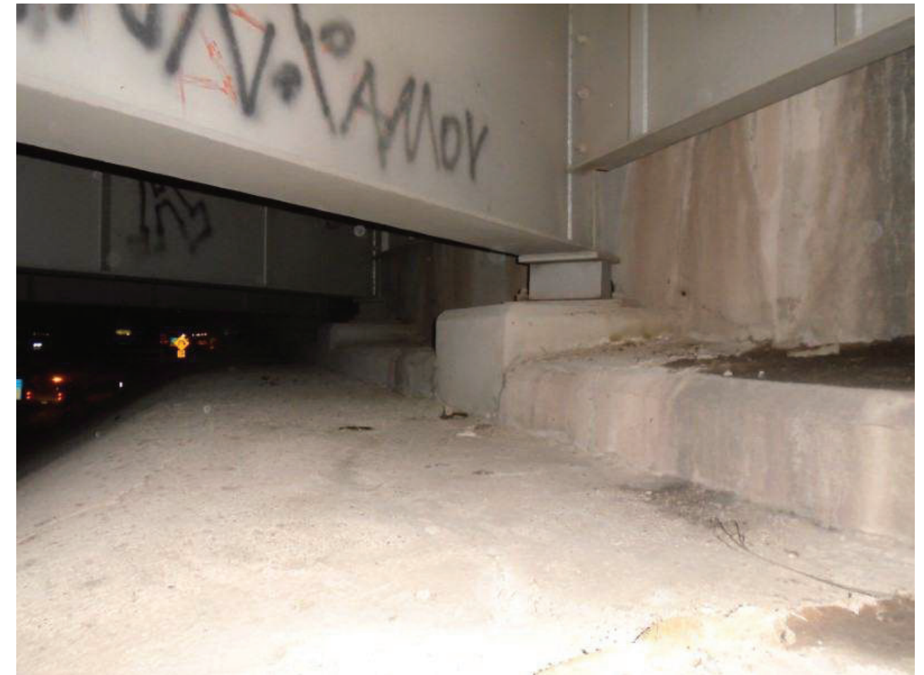
File Name : 01214-2020-05-31-Photo-11.JPG Description : North Abutment, LNE
