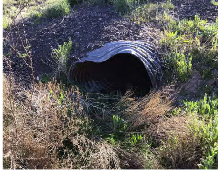
CULVERT #100 INLET 36" X 22" CMP ARCH STA 1050+00
