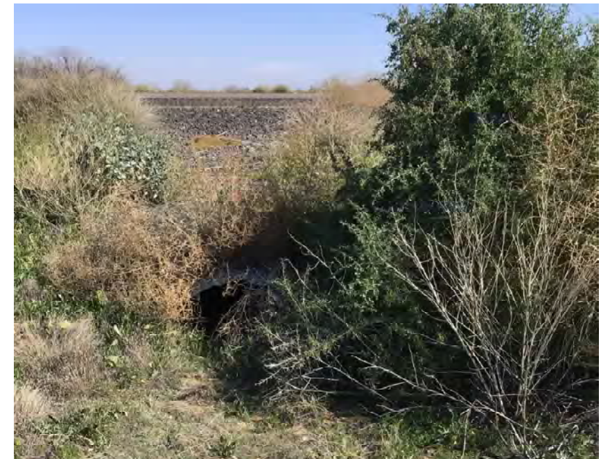
CULVERT #175 OUTLET 36" X 22" CMP ARCH STA 1136+50
