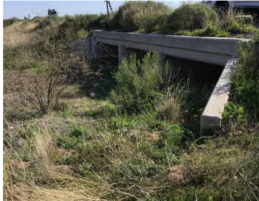
CULVERT #215 INLET BOX CULVERT 3- 10' X 3' STA 1202+02
