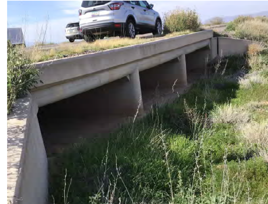
CULVERT #270 INLET BOX CULVERT 3- 10' X 3' STA 1253+00
