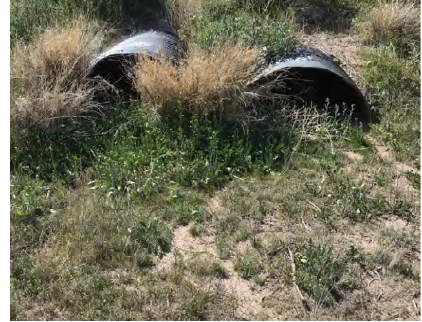
CULVERT #415 INLET (2) - 43" X 27" CMP ARCH STA 1429+00
