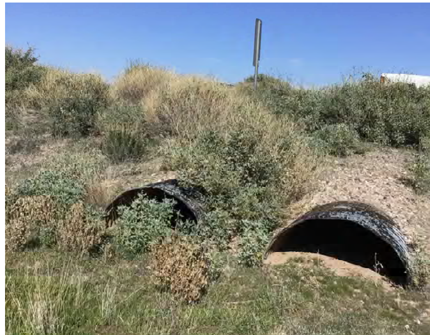
CULVERT #265 OUTLET (2) - 43" X 27" CMP ARCH STA 1249+00
