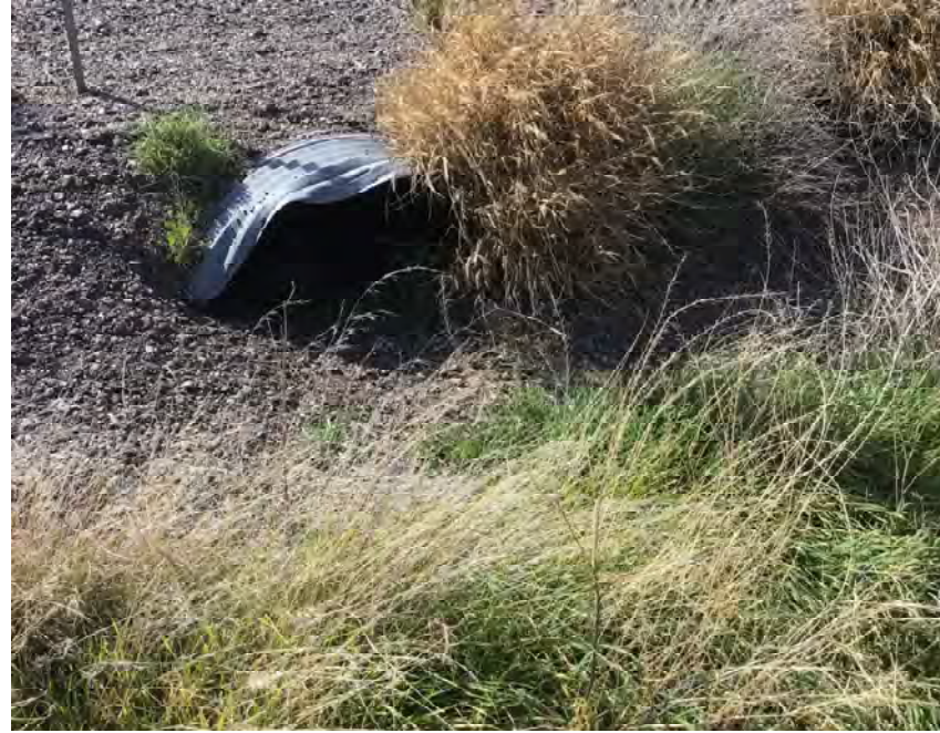
CULVERT #305 INLET (2) - 43" X 27" CMP ARCH STA 1291+00
