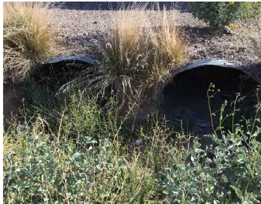
CULVERT #305 OUTLET (2) - 43" X 27" CMP ARCH STA 1291+00
