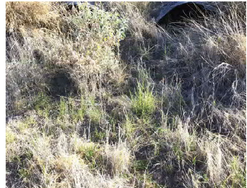
CULVERT #290 OUTLET (2) - 43" X 27" CMP ARCH STA 1273+00
