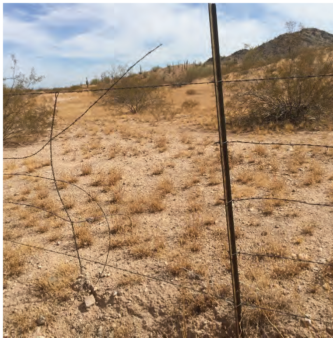
Figure 1. Damage to fencing along I-10.
