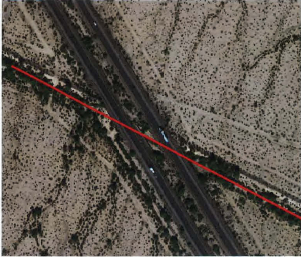
Figure 9: Southside Levee and six barrel box culvert.
