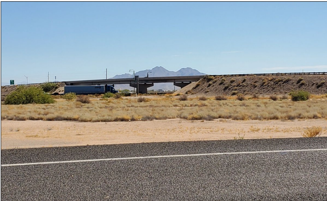
Figure 3. Typical view of a freeway bridge
