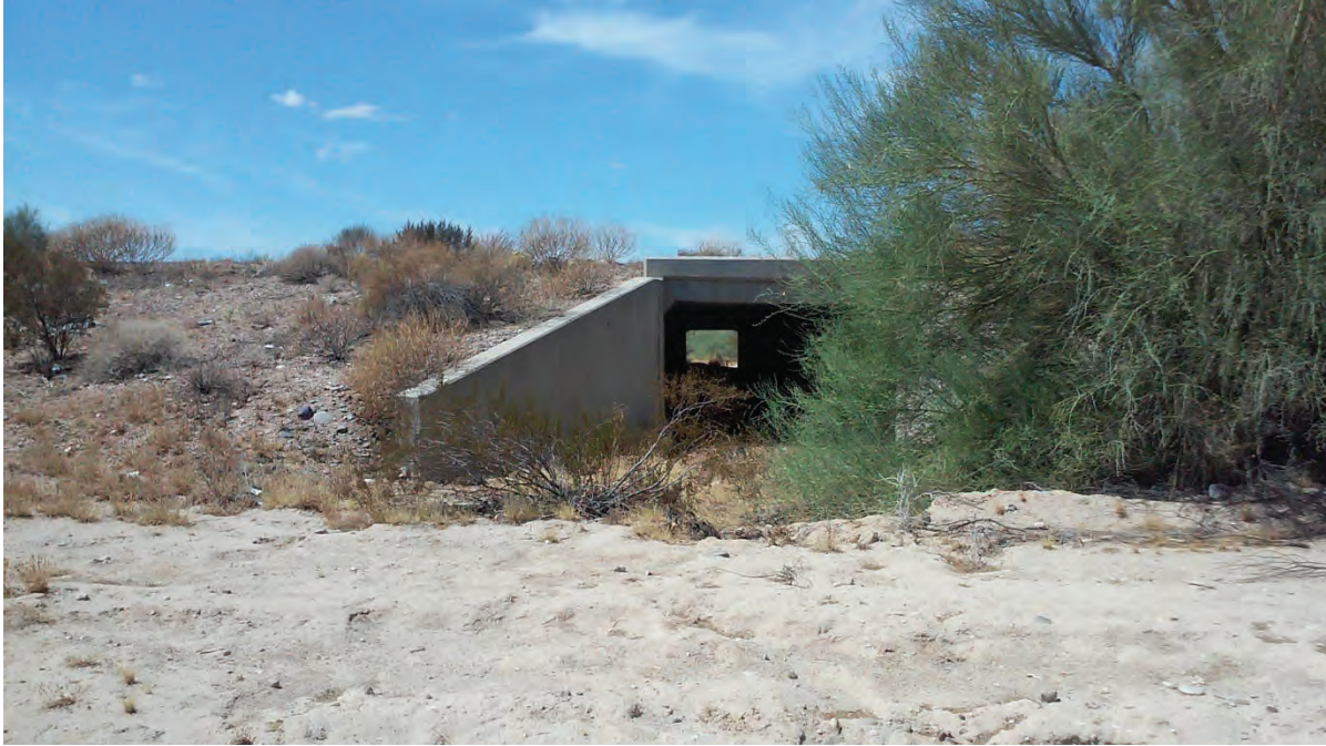
Figure 5. Culvert with an evident exit route visible to crossing wildlife.
