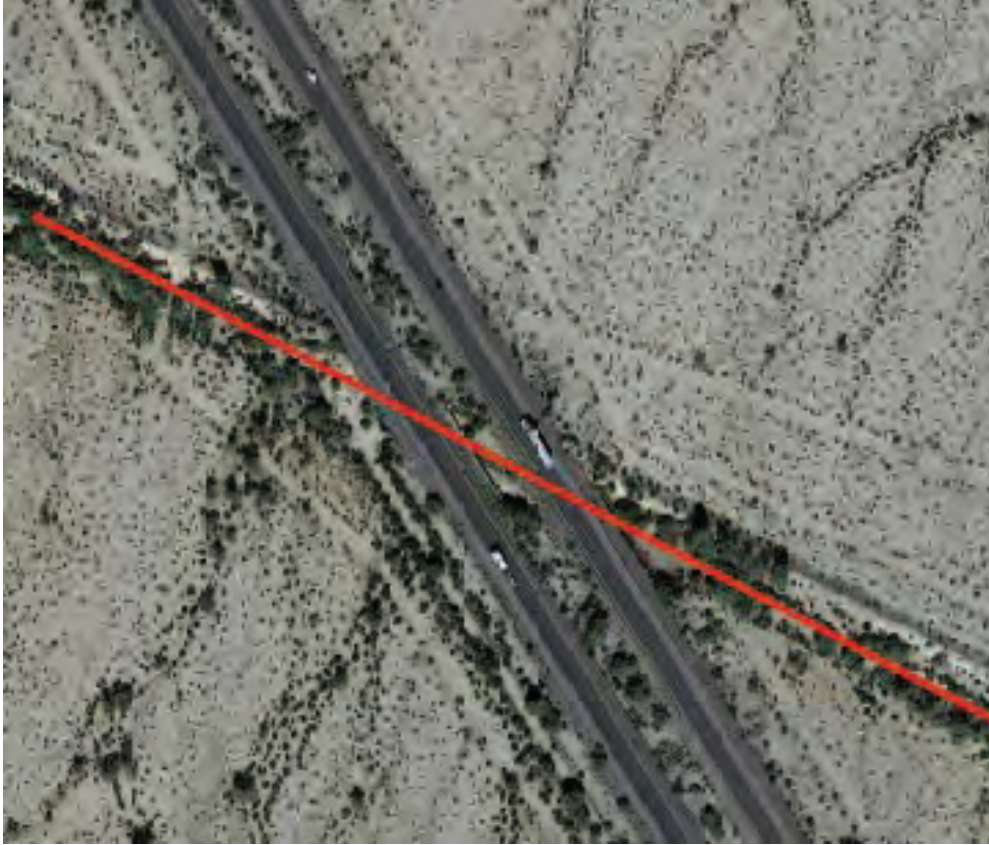
Figure 9: Southside Levee and six barrel box culvert.
