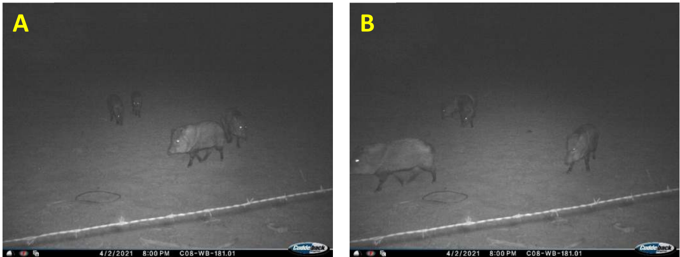
Figure 4. Photo A shows javelina approaching the WB opening of Culvert C08 and Photo B taken approximately 5 seconds later show the javelina being repelled from the structure rather than using it to cross under I-10.
