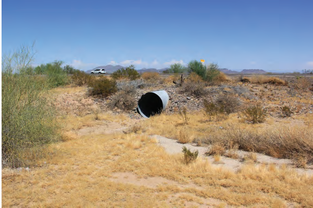
Figure 3. Corrugated metal pipe which spans the entire length across Interstate 10.
