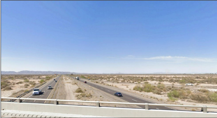
Figure 20. View north from Riggs Road overpass
