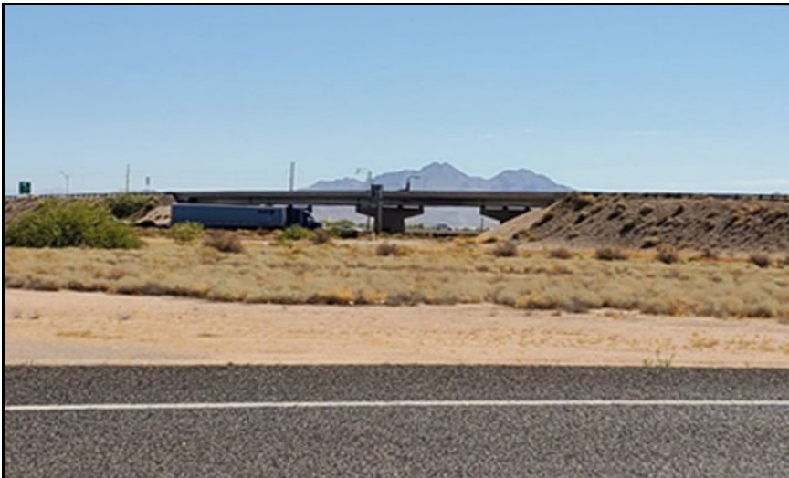
Figure 22. Typical view of a freeway bridge
