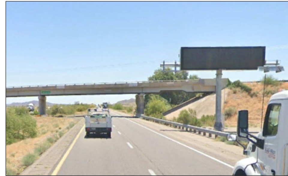
Figure 1-3. Dynamic message sign along eastbound I-10, Sta 1805+60, on butterfly structure approaching Seed Farm Road
