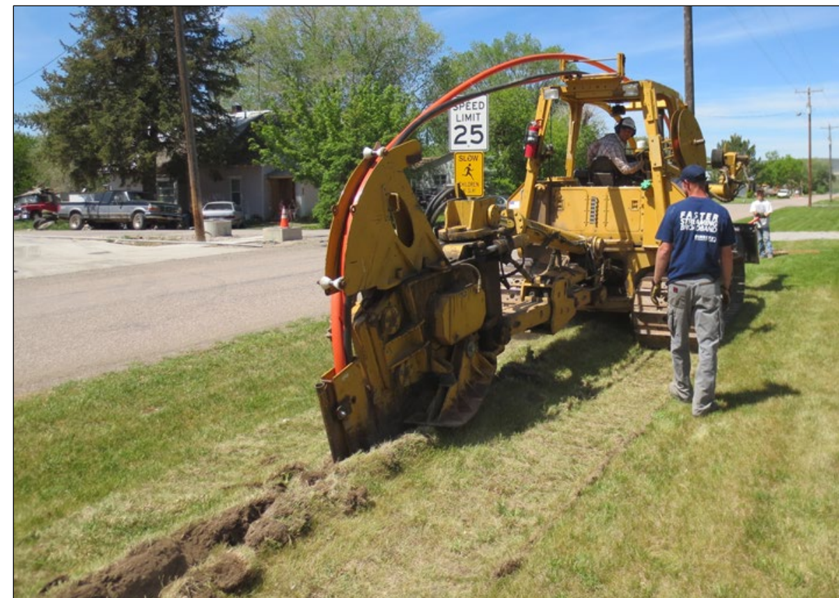
Figure 3-33. Sample fiber optic plowed installation
