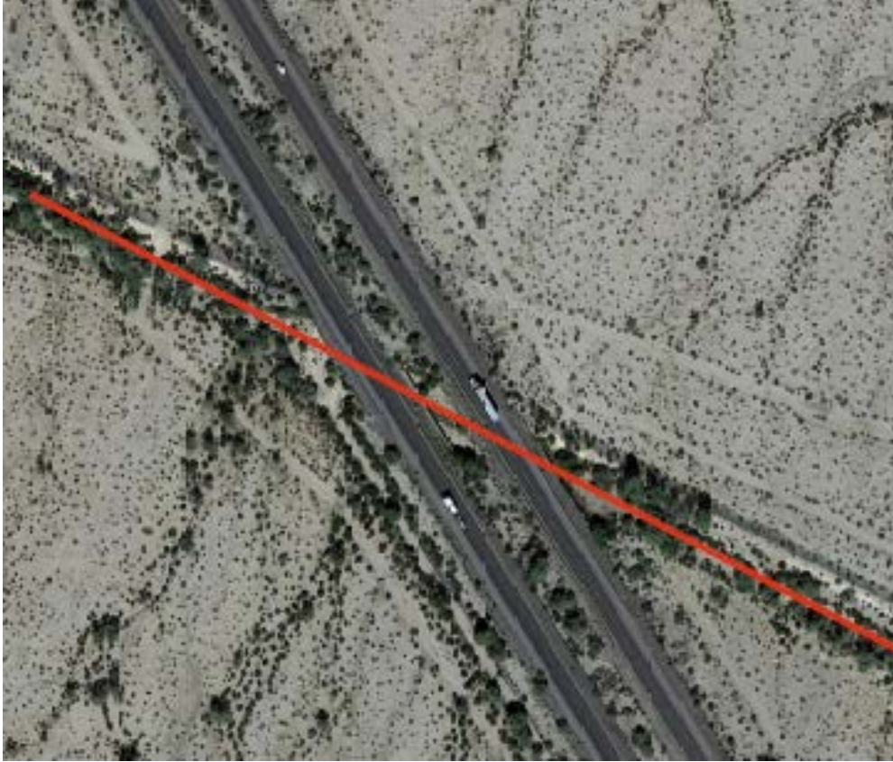
Figure 9: Southside Levee and six barrel box culvert.
